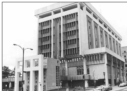
District One / Police Administration Building 749 West State Street, Milwaukee, WI 53233
