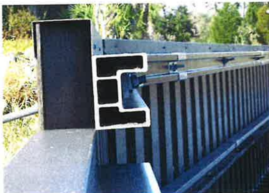
Example of composite bulkhead, wale, and cap with hot dipped anchor tie rods.
