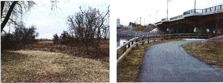
(Left) View to existing wetland looking north; (Right) New underpass trail at Route 16 bridge.
