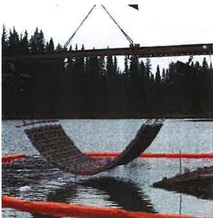
Example of the installation of articulated block mats at a boat launch.
