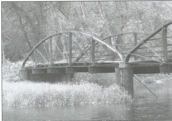
Photo credit: Friends of McGilvray Road. Bridge 4
