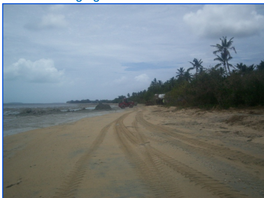
Dredging of fine sand at 5 m from LWM.
