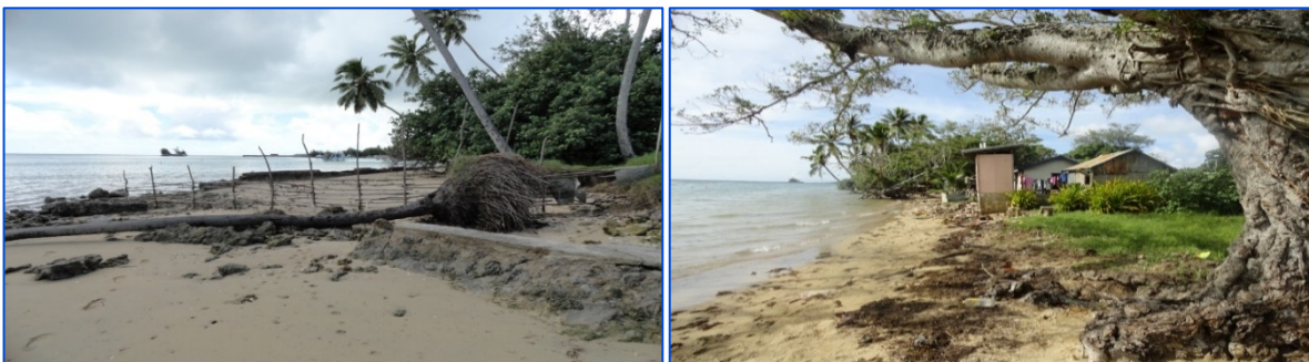
Severe erosions at Lifuka Island.
