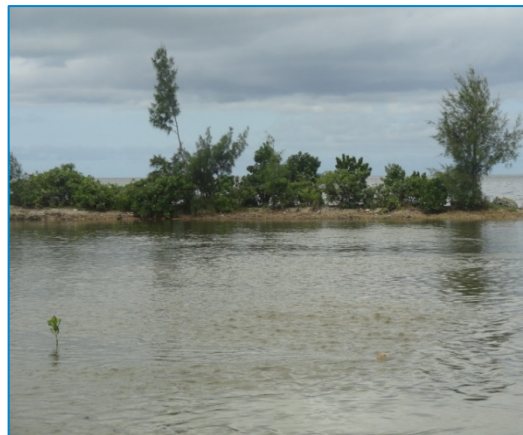
Showing no vegetation regrowth where there is behind the breached in the rock revetment.
