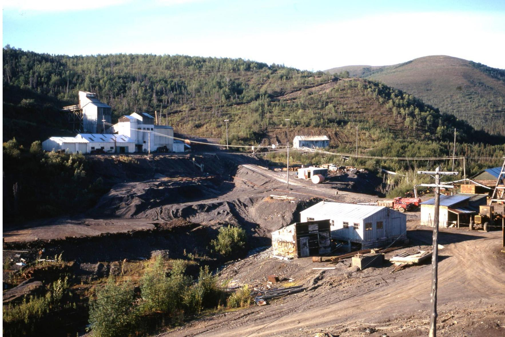
Main Processing Area in 1969, showing the flotation mill (left) added to the post-1955 processing building, and the settling ponds.
