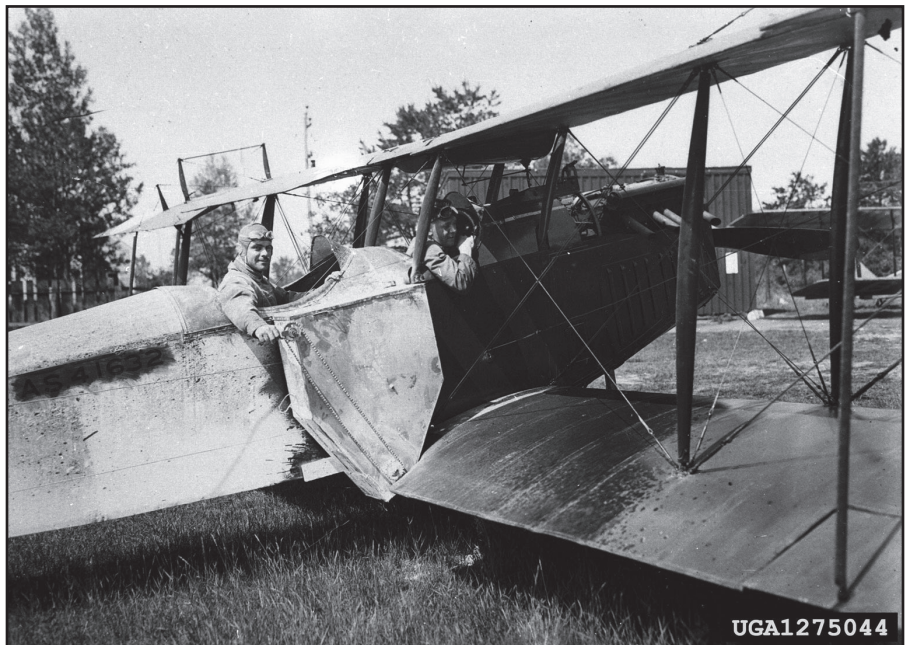
Figure 6-1. Early aerial gypsy moth treatments were manually released.
