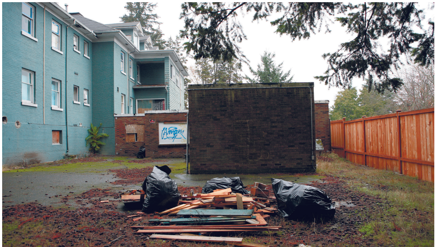
CP8. Looking north along east side of property.
