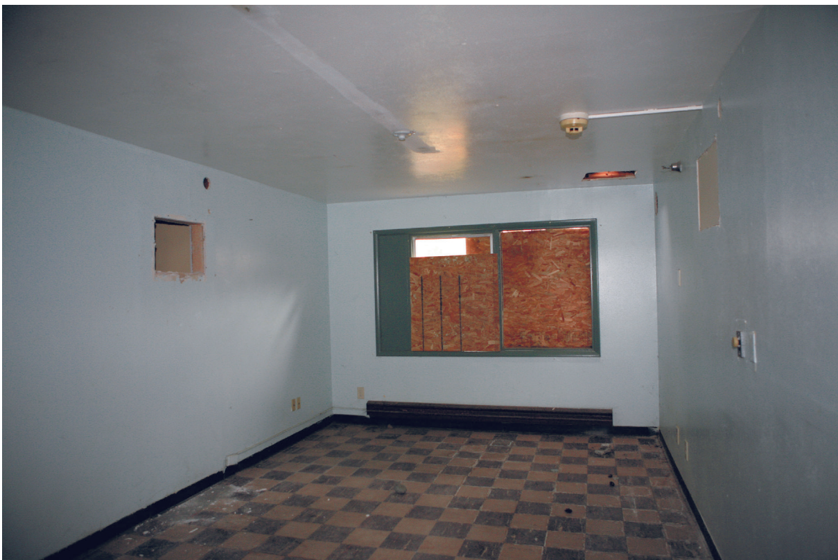
CP24. Basement (Annex), typical room.
