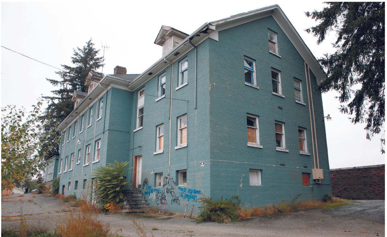
CP6. Southwest corner.
