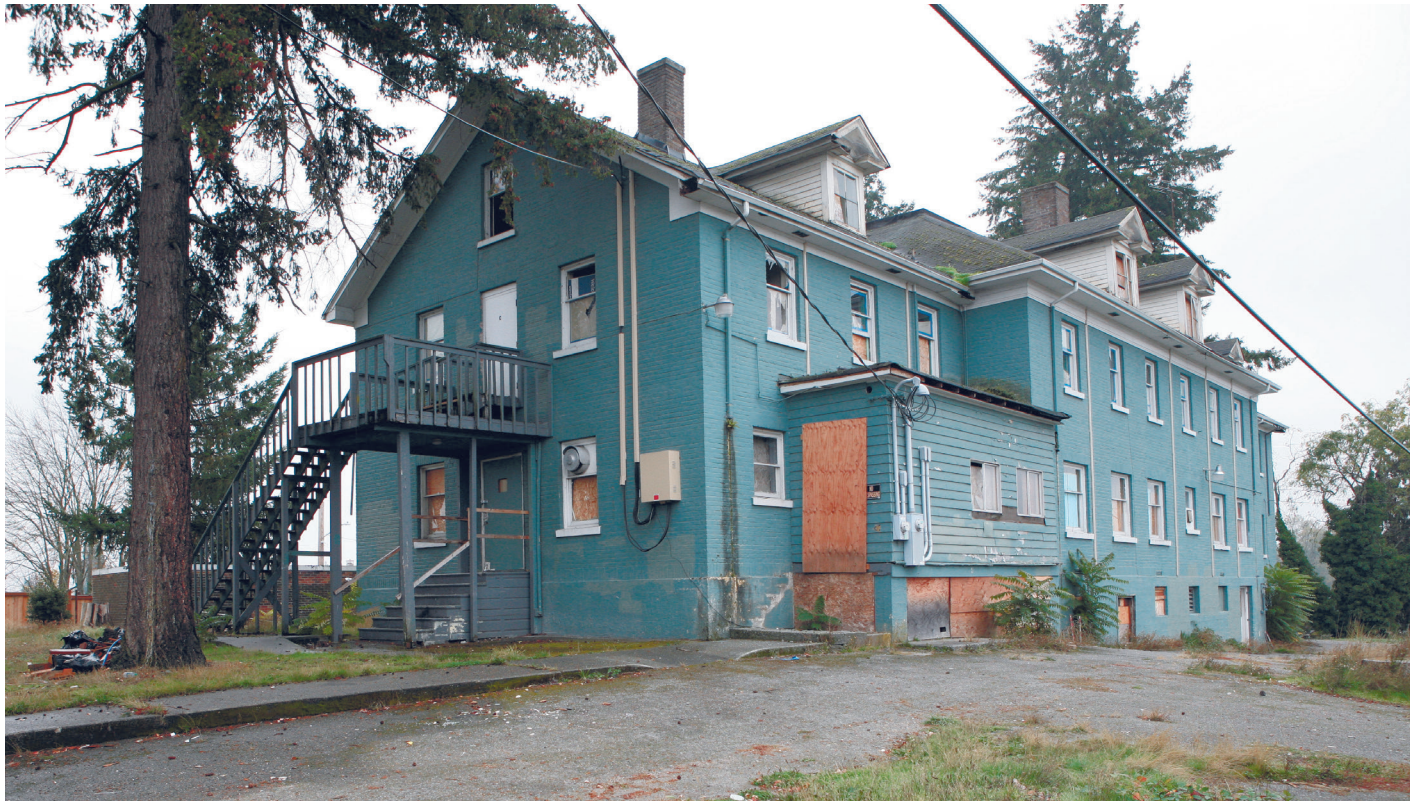
CP4. Northwest corner.
