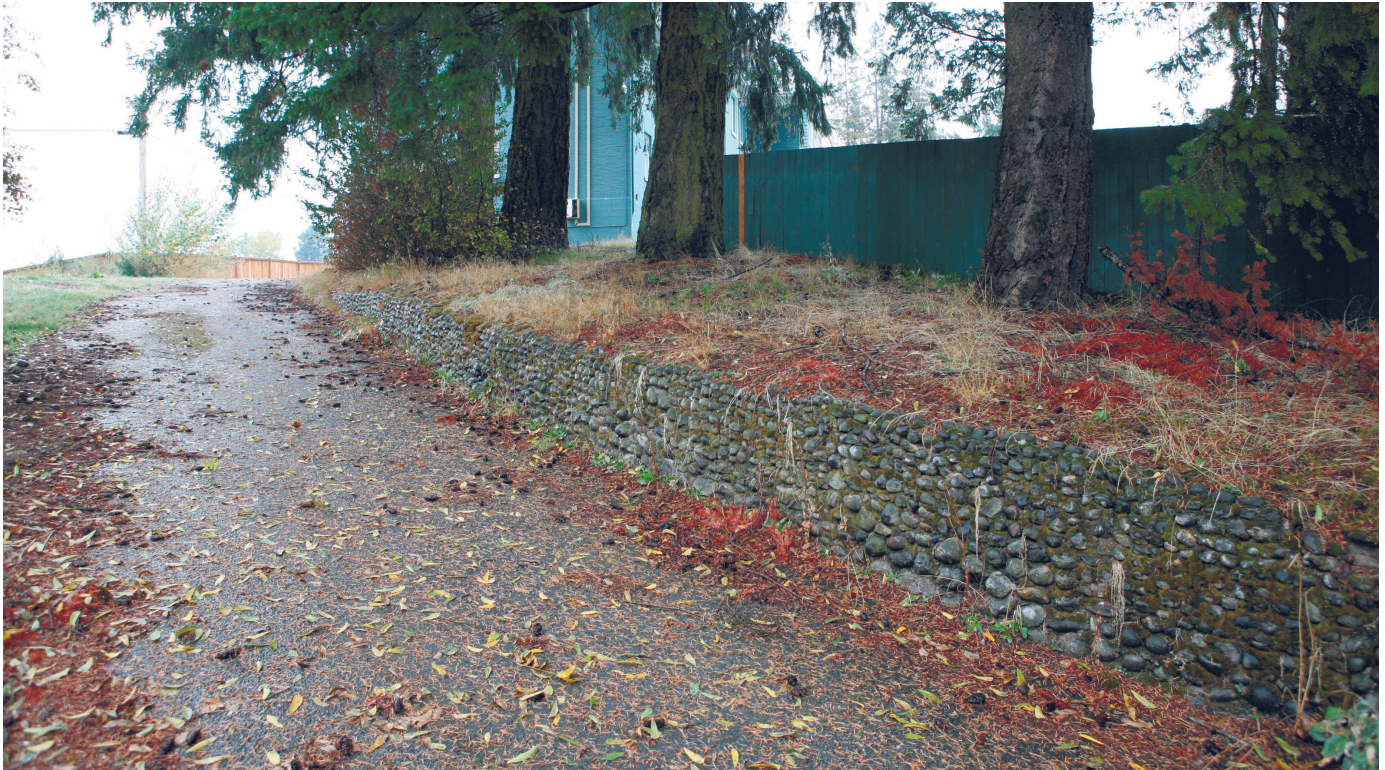
CP9. River rock retaining wall, paved driveway along south south side of property. Looking northwest.
