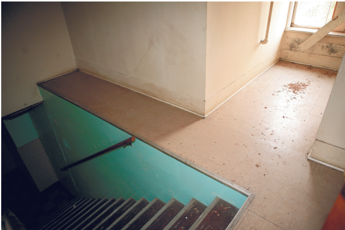
CP20. Top of stairs to attic.
