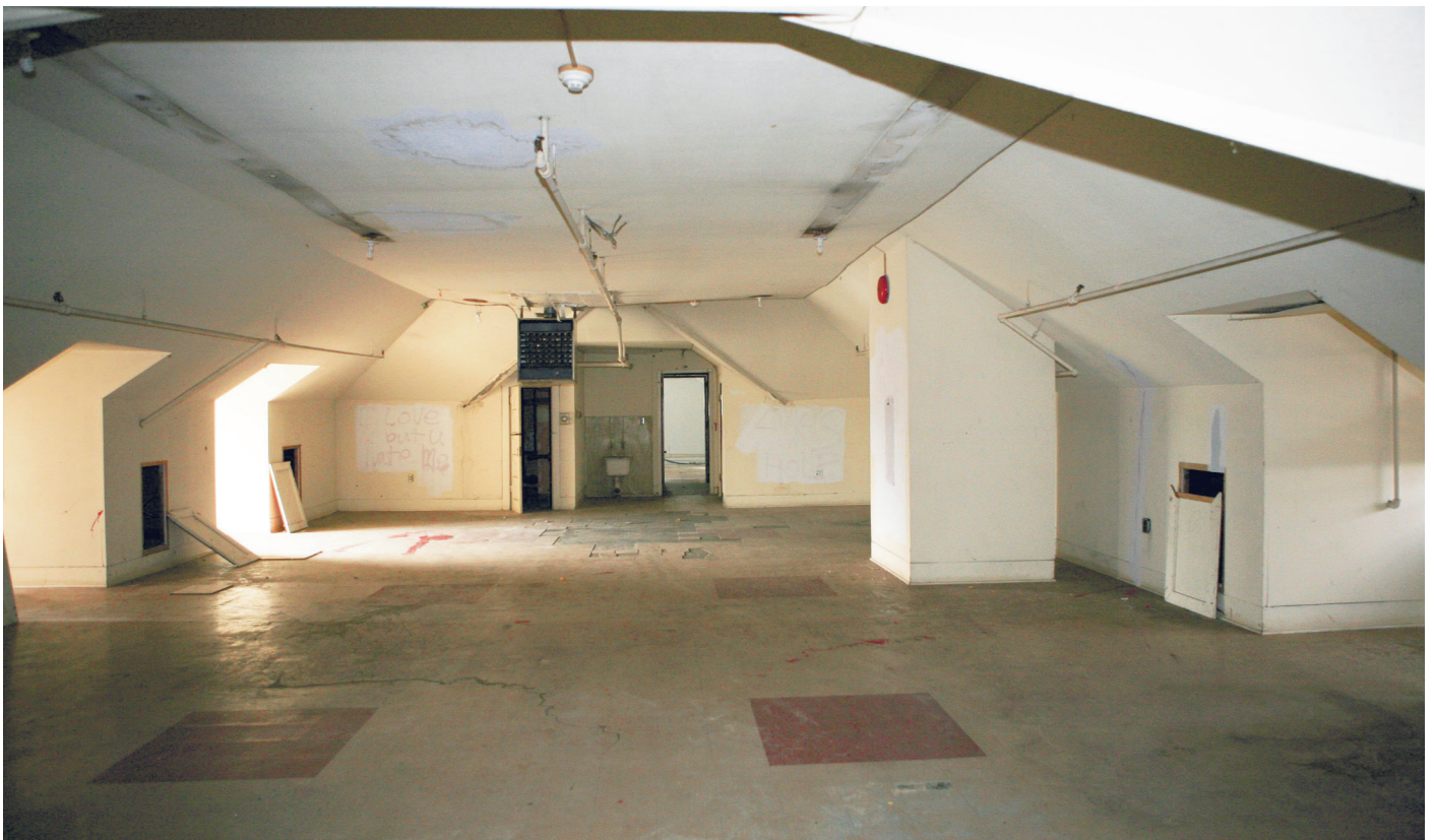
CP22. Attic, looking south.
