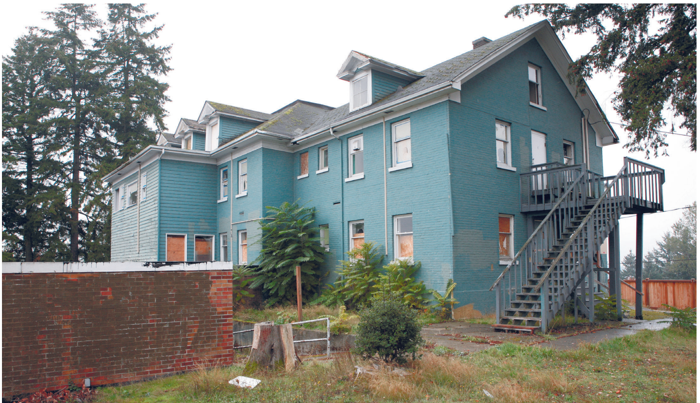
CP2. Northeast corner. Low brick addition at left.
