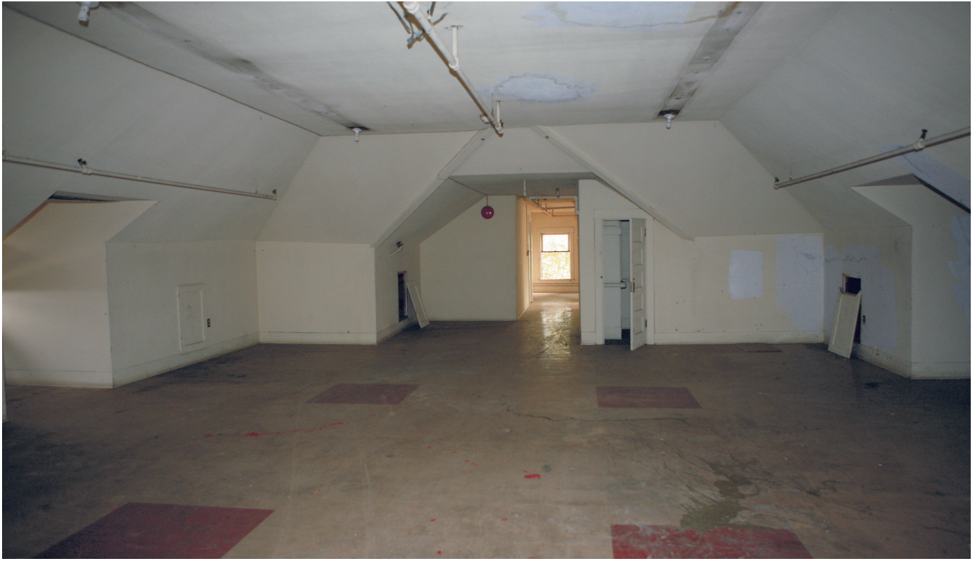
CP21. Attic, looking north.
