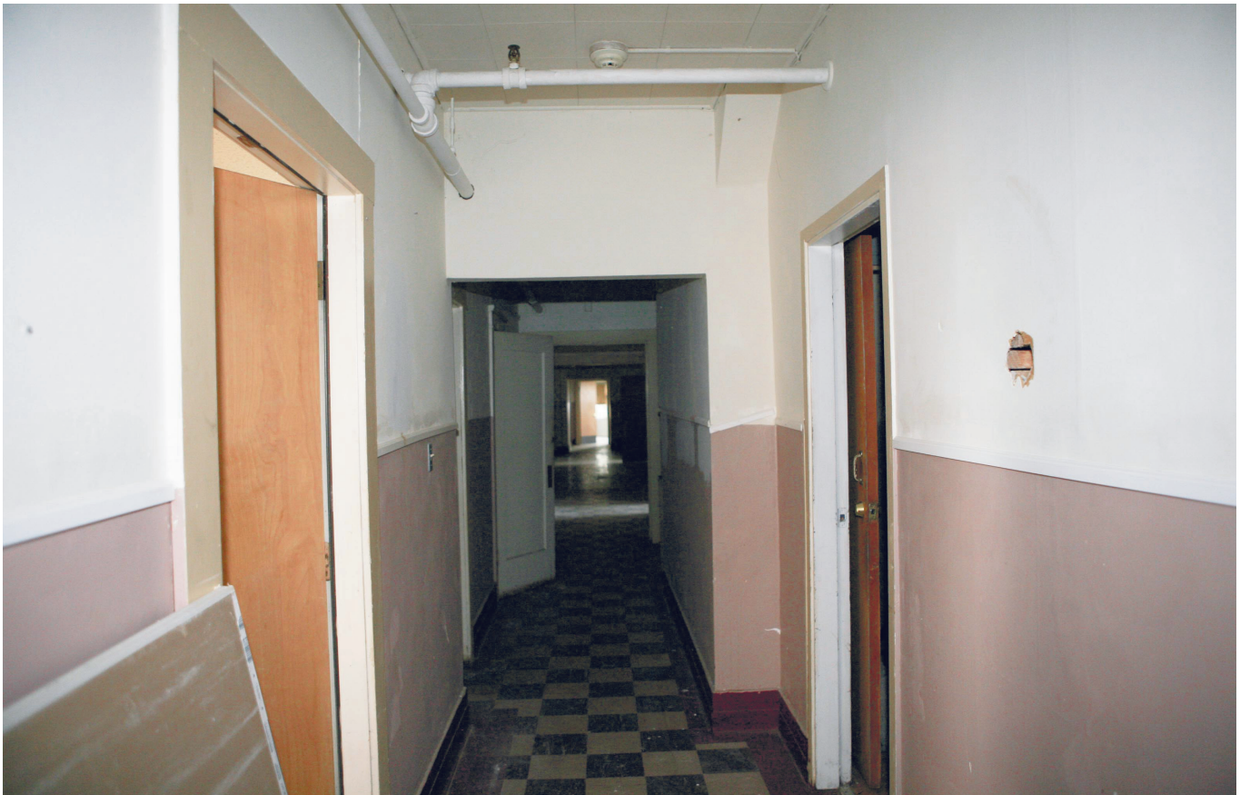
CP10. First floor corridor, looking south from north entrance.
