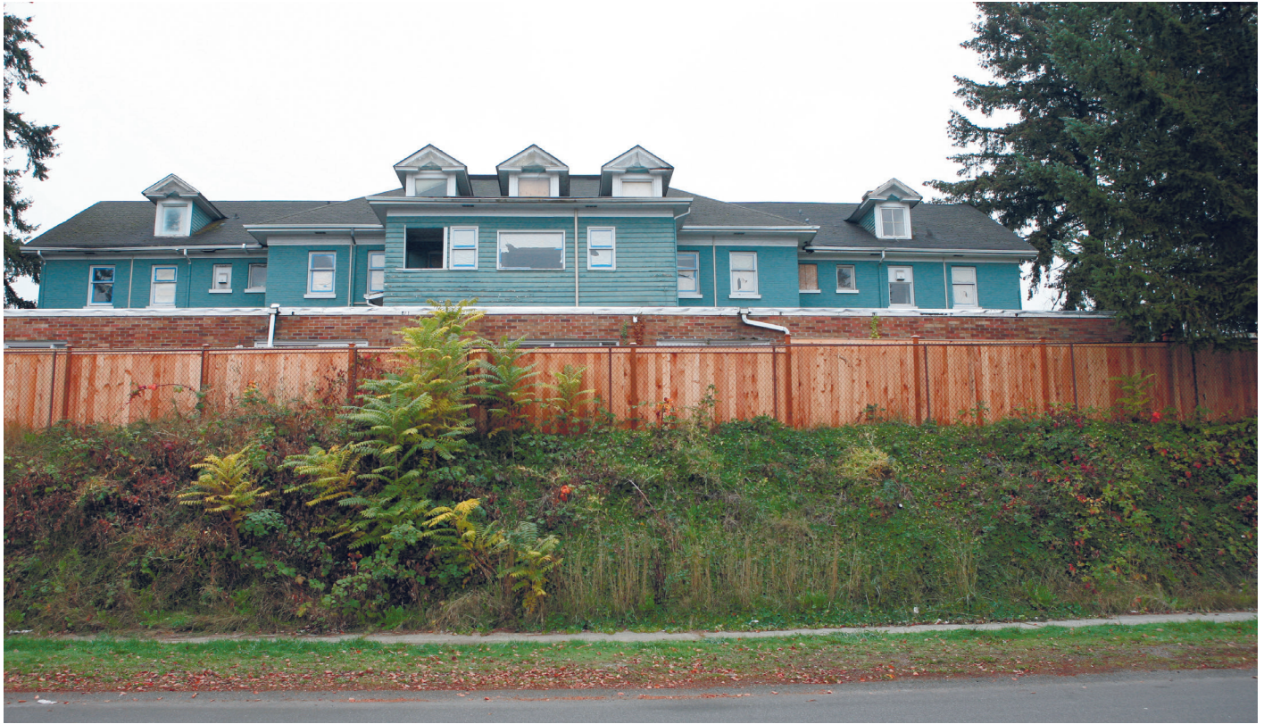
CP1. Front (E) facade, from S. State St.
