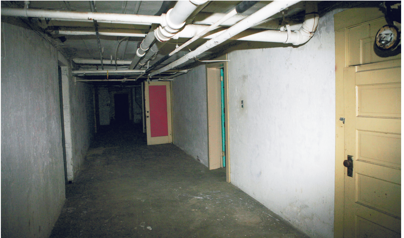
CP23. Basement, main building.
