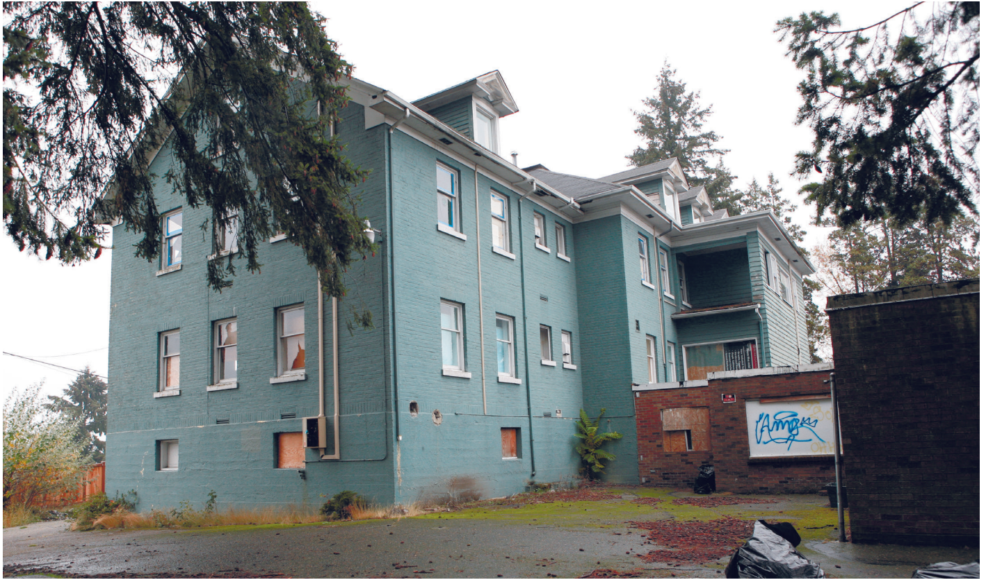
CP7. Southeast corner. Low brick addition at right.
