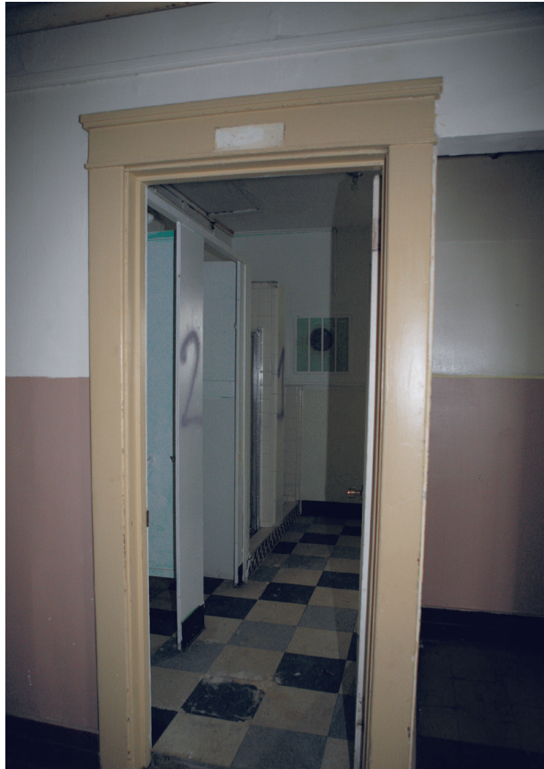
CP12. First floor, looking west from main corridor into multi-stall restroom.
