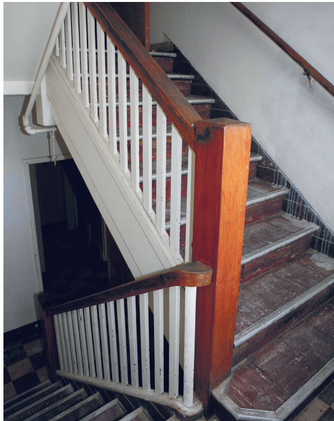
CP14. First floor, stairwell, west side of main corridor.
