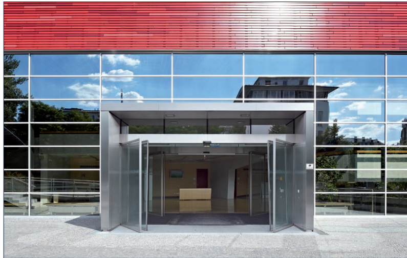
Rechts der Isar Hospital of the Technical University of Munich, Germany (Photo: Robert Sprang)
