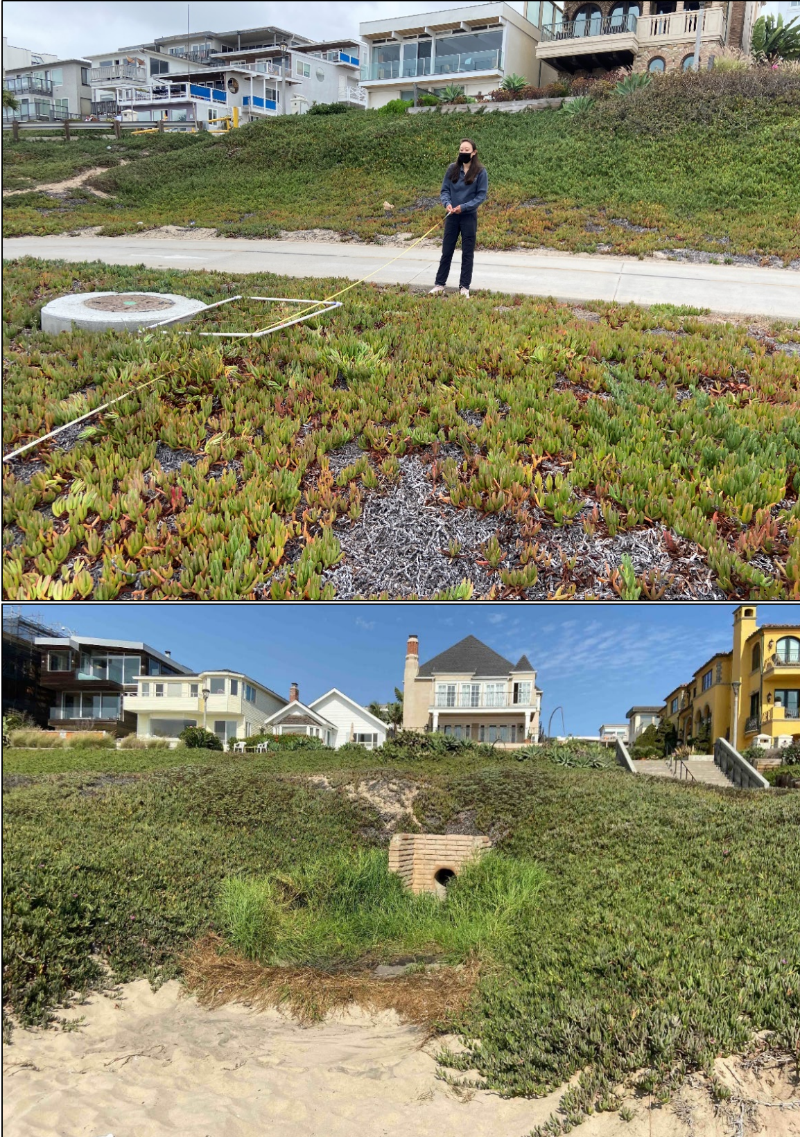
Figure 11. Photos showing one of the seven maintenance holes within the project area (top) and one of the two outfalls adjacent to the area (bottom).
