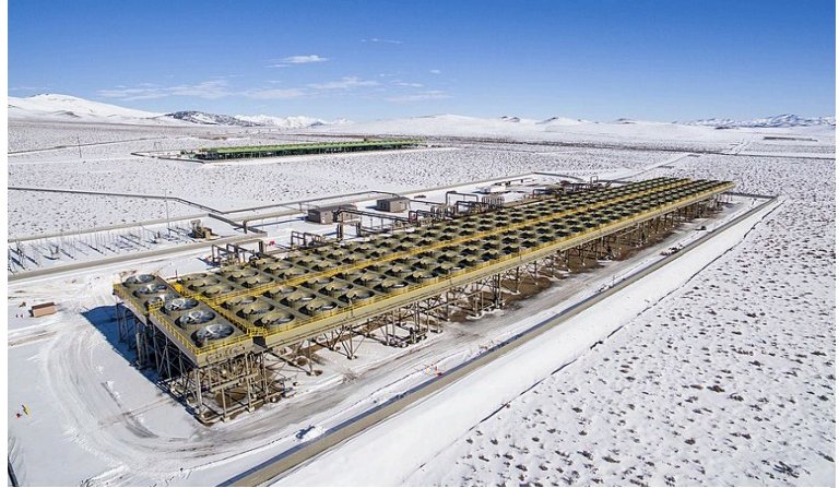
McGinness Hills Geothermal Plant | Source: Nevada BLM
