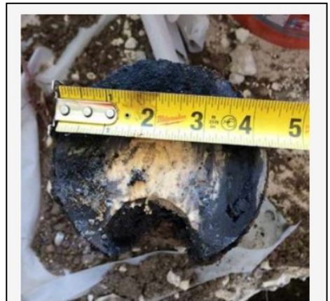
Figure A – Top view of a section of 4 inch cast iron pipe from a condominium experiencing severe FOG buildup.
