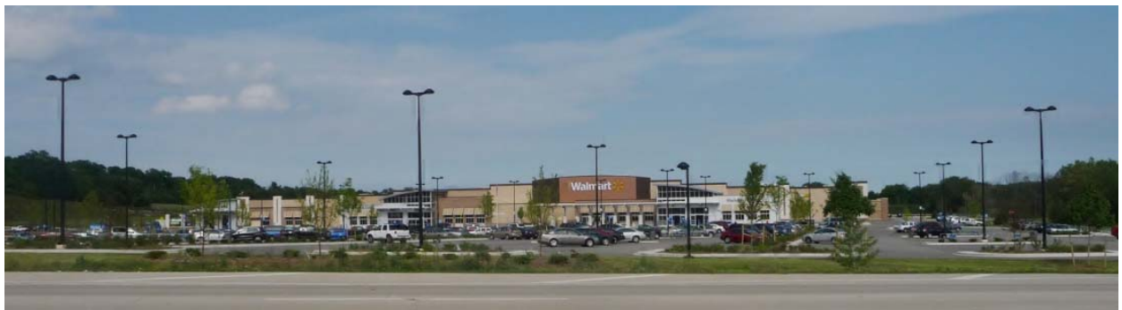
Wal-Mart is one of three new regional retailers to locate along the east side of Moorland Road.
