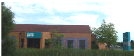
Single tenant and auto-oriented commercial structures are common features along Janesville Road.
