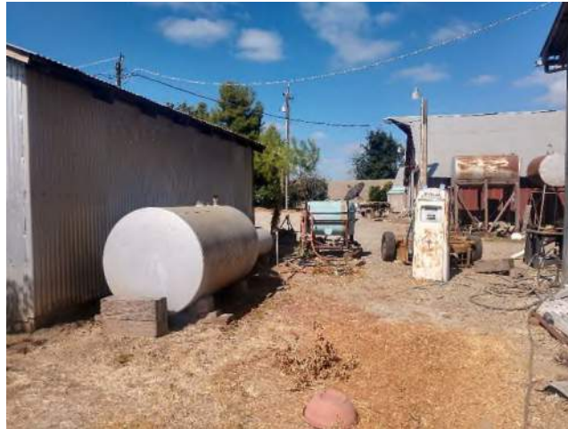
Figure 5 – View of AST and gas dispenser.
