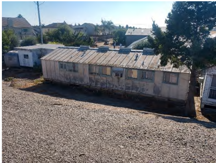
Figure 14 – View abandoned “barracks” structure.
