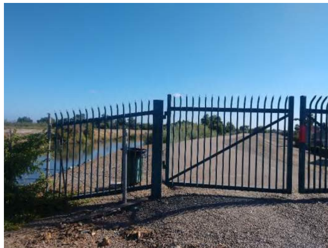
Figure 18 – View of northwest boundary of site, looking north.
