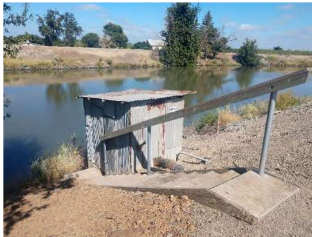
Figure 20 – View of river inlet piping (pump station?) facing west.
