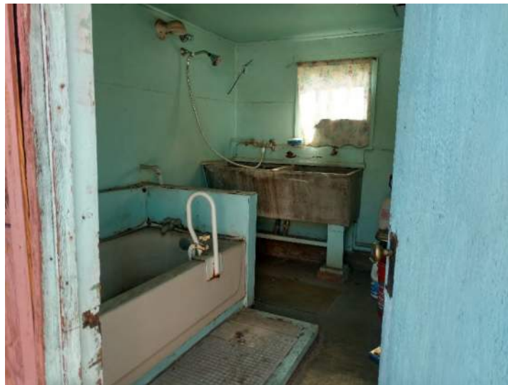
Figure 9 – Inside view of bath house.
