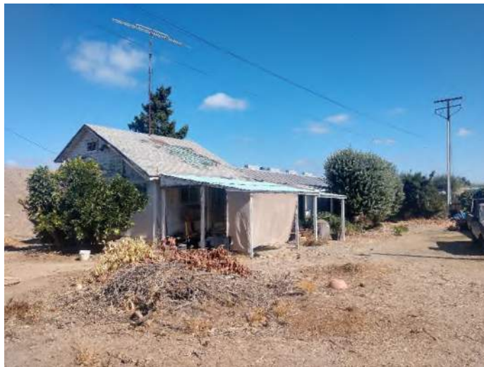
Figure 15 – View of abandoned house structure facing northwest.
