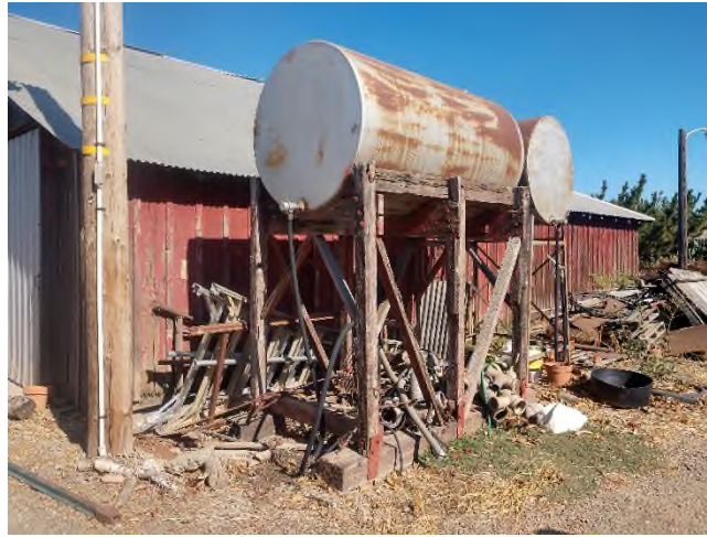
Figure 3 – View of two ASTs adjacent barn.
