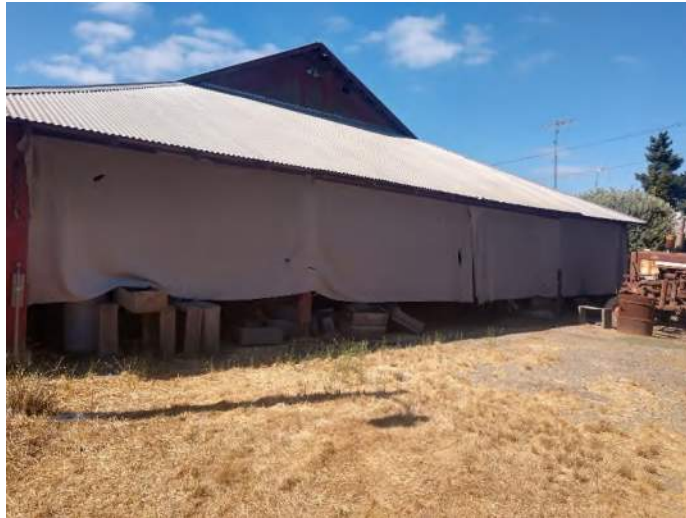
Figure 11 – View of barn facing south.
