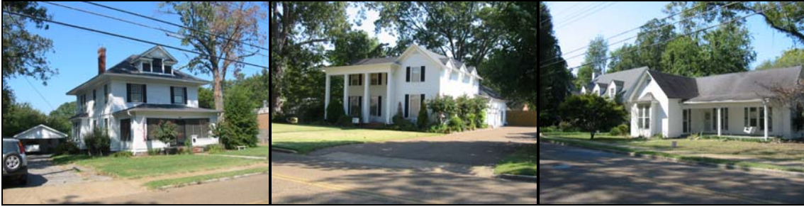
Representative dwellings within the South College Historic District.
