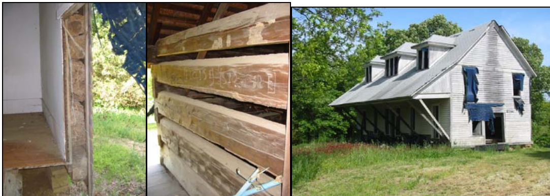
Wiseman-Overall House (TP-273) located at 6422 Highway 59 in Burlison.
