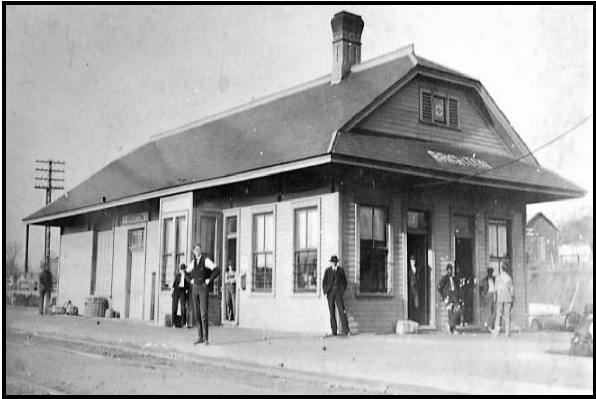
Brighton Depot built in 1903 and shown here ca. 1905. Passenger and freight depots were the centers of railroad communities such as Brighton. The building is currently still extant (Source: TSLA).
