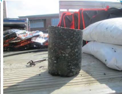
CORE 9 150' N of Spruce St.; 3' off W curb
