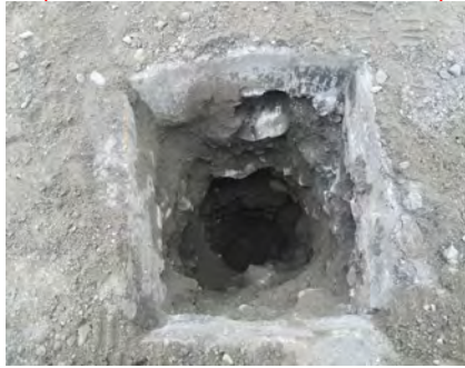
TEST PIT 11 50' N of Mulberry St.; 4' off W curb
