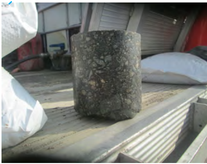
CORE 1 150' S of Everett City Line; 5' off W curb
