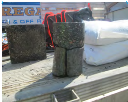
CORE 15 140' S of Chestnut St.; 5' off E curb
