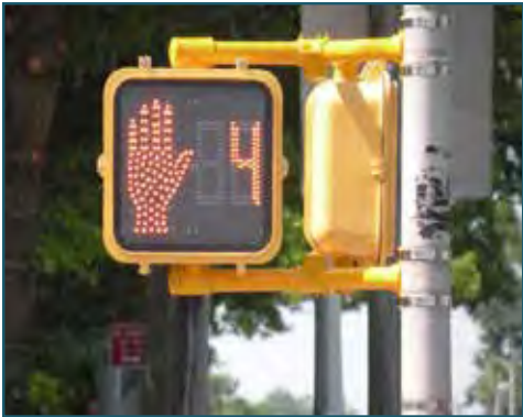
Pedestrian Countdown Signal Head
