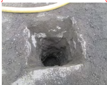
TEST PIT 8 450' N of Spruce St.; 6' off E curb
