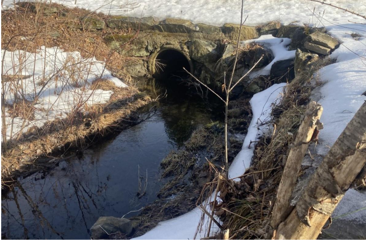
Washington St. Culvert
