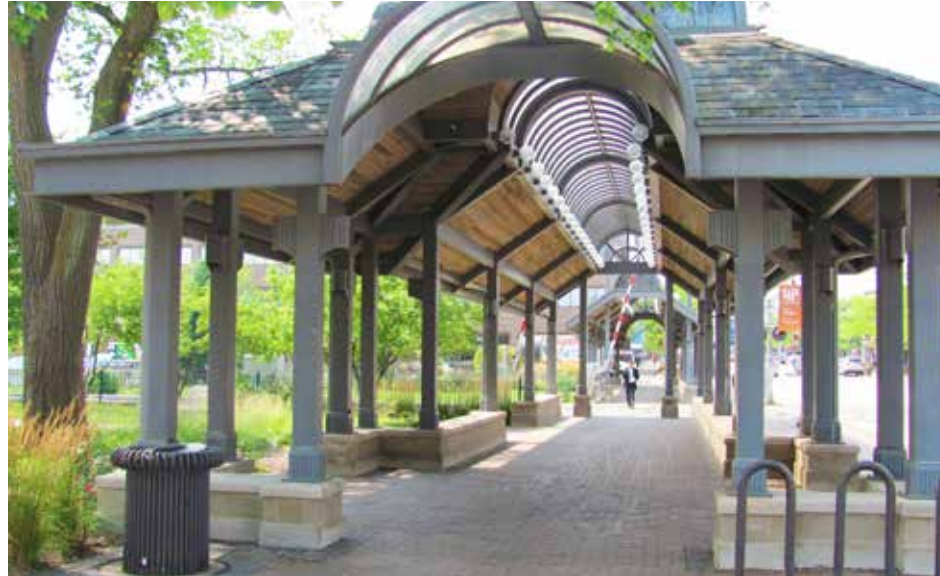
Streetscape. Pedestrian Arcade
