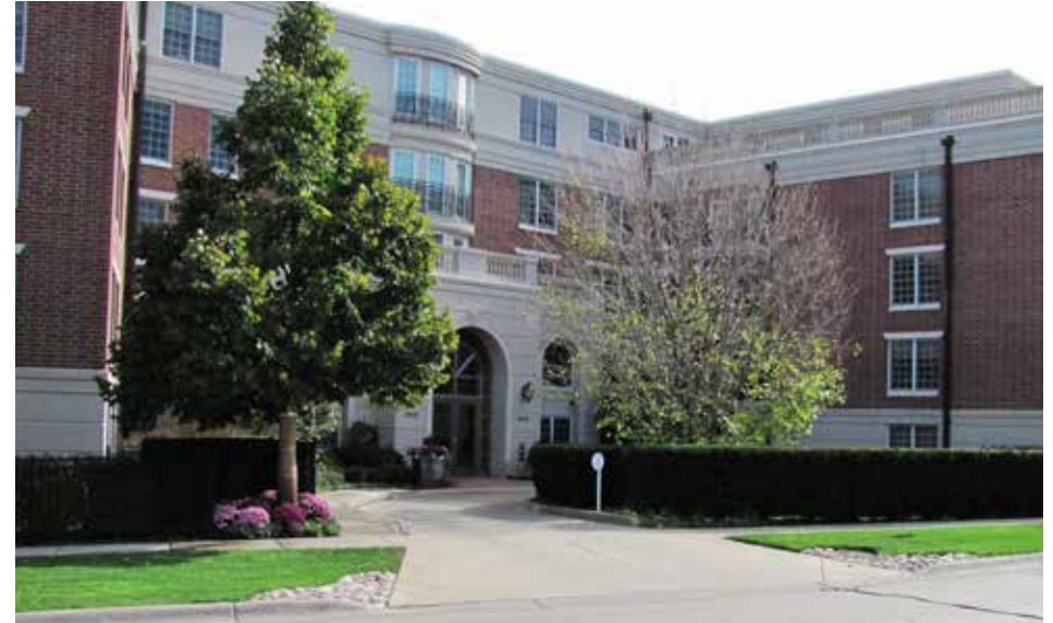
Building Bulk. The bulk of a building can be broken up with horizontal exterior design features and upper story setbacks like this building located along St. Johns Avenue
