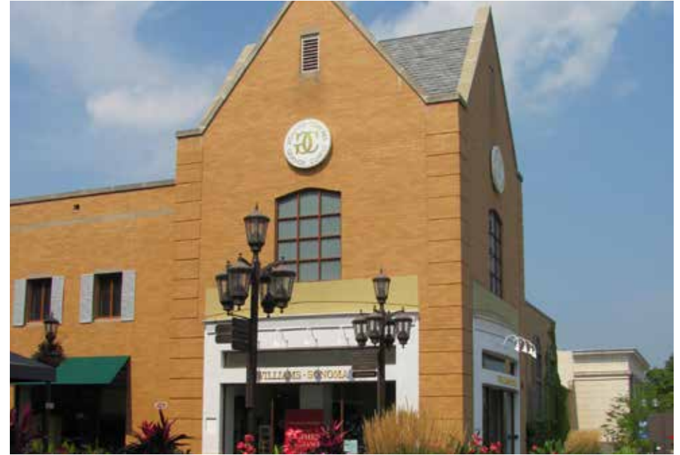
Corner Lots. Building design takes advantage of corner lot with change in roof line and shorter setback along Second Street
