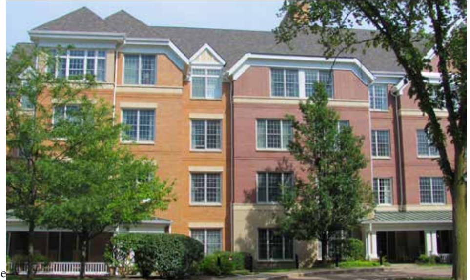
Building Bulk. Variation in brick color creates the illusion of two different buildings, lessening the apparent bulk of the building located along Green Bay Road
