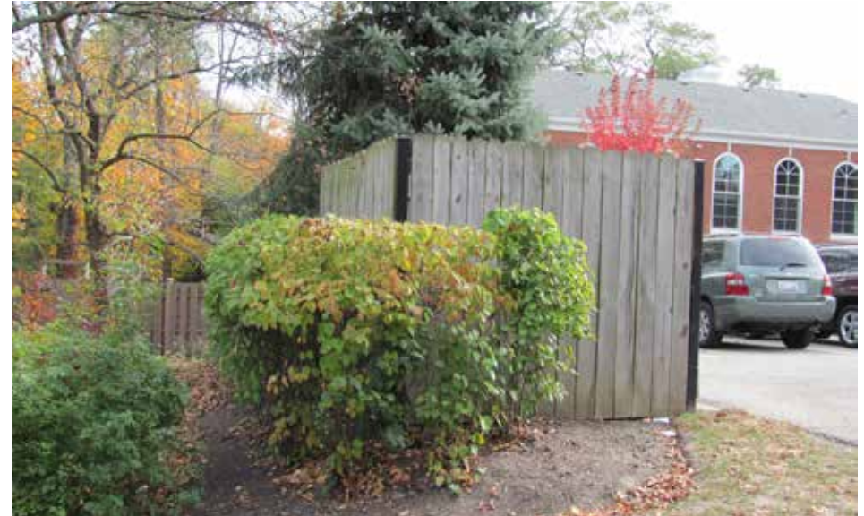
Mechanical Screening. Equipment is screened with both fencing and landscaping behind City Hall
