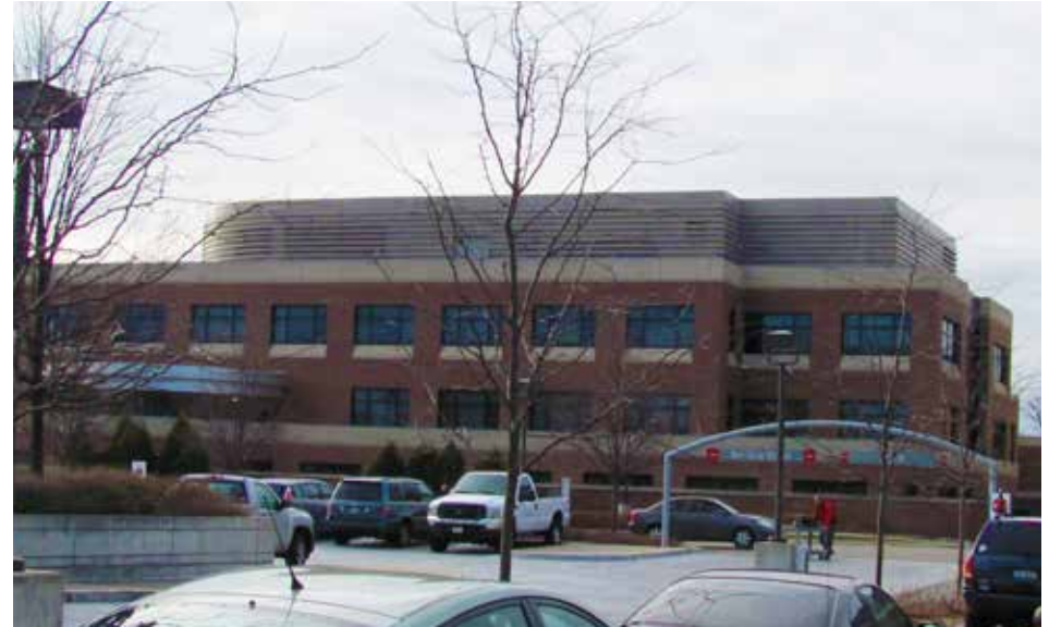
Roofing. The design includes screening of mechanical equipment on the roof of Highland Park Hospital building.
