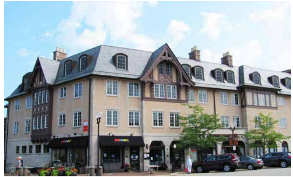
Building Bulk. Bulk is broken up with change in exterior building materials, vertical elements, and change in roof line of building located at the corner of Park Avenue and Sheridan Road
