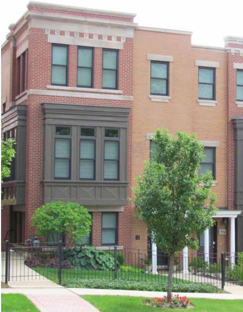
Building Bulk. Change in materials and varying building setback break up mass of building located along Laurel Avenue
