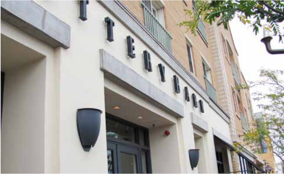
Lighting. Lighting fixture color matches the color of sign lettering along Second Street
