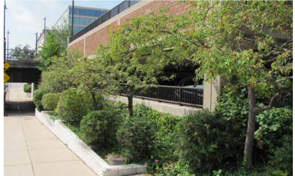
Parking Structure. Landscaping screens the parking structure along Laurel Avenue from the public right-of-way
