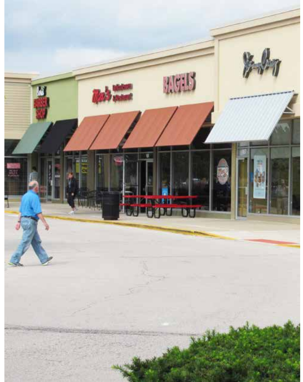
Awnings. Awnings on businesses at Crossroads Shopping Center
