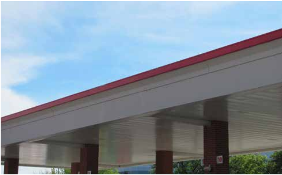
Lighting. Gas station located along Skokie Valley Road uses recessed lighting under structure that blends into white material of the structure and LED lighting above
