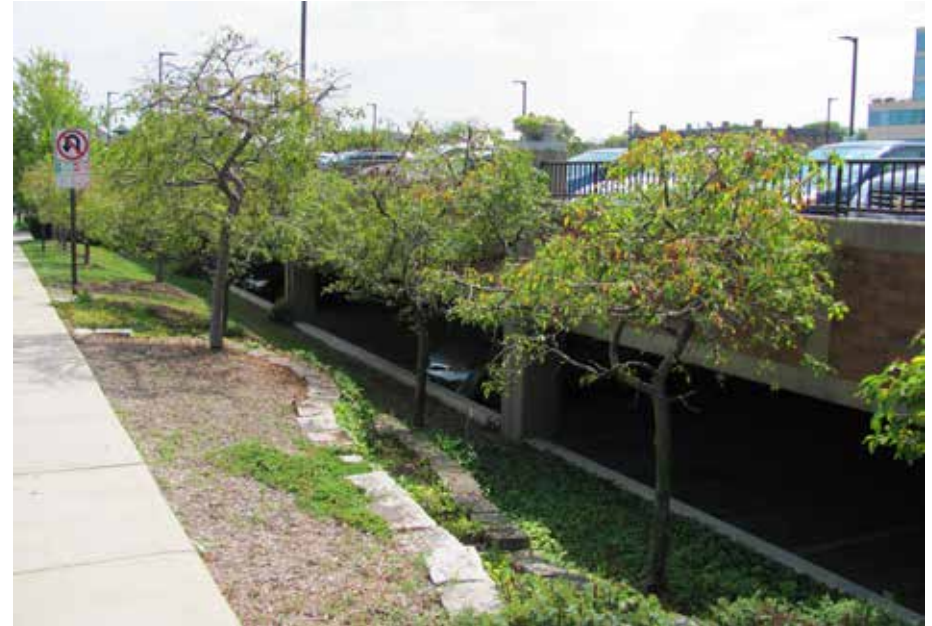
Parking Structure. Parking structure located along St. Johns Avenue incorporates landscaping into the design. (See Article 22 of Chapter 150 of the Municipal Code for details)
