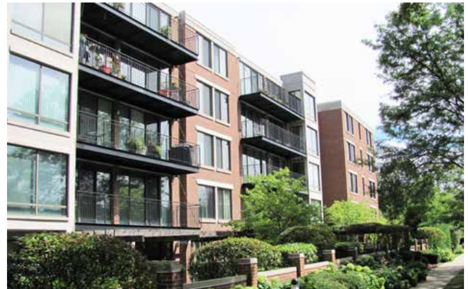
Building Bulk. Change in materials, protruding masses, and balconies break up mass up building located at the corner of Second Street and Walnut Street
