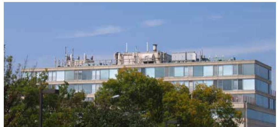
Antennae. Rooftop telecommunication antennas on First Street and Laurel Avenue
