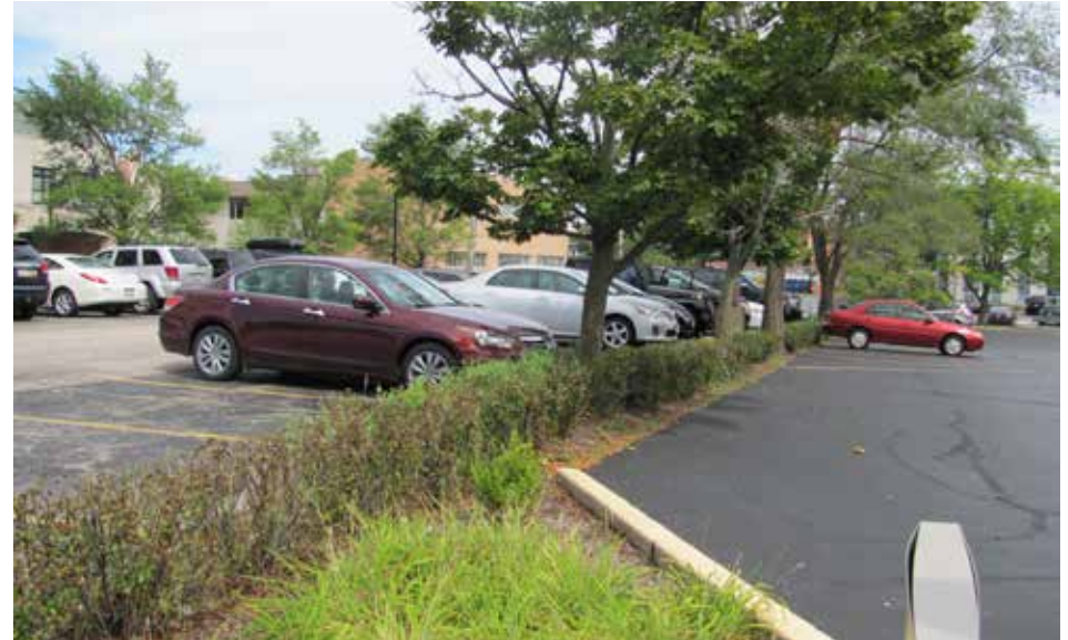
Parking Lot Landscaping. Landscaping is used to separate two parking lots located along St. Johns Avenue
