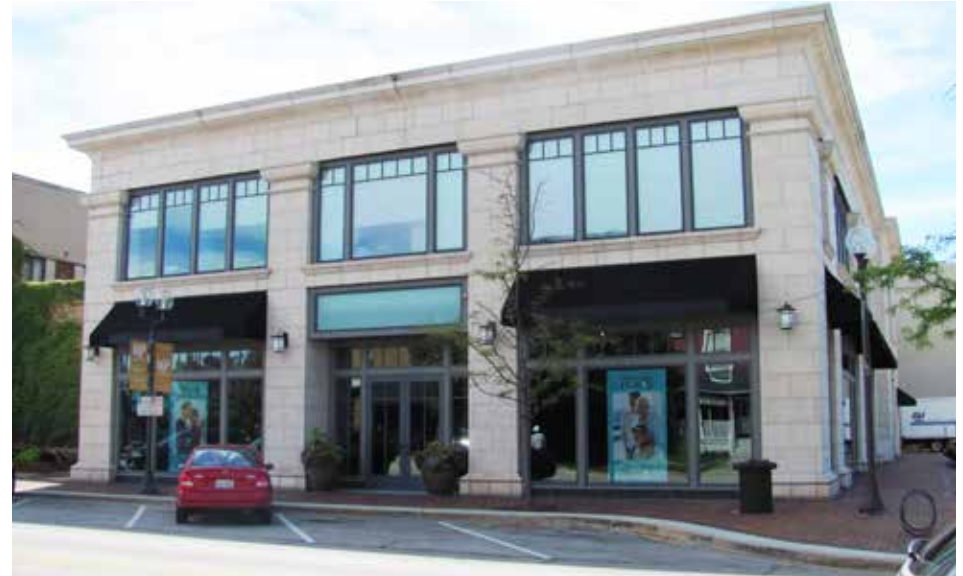
Building Material and Facade Example. Building along Second Street
