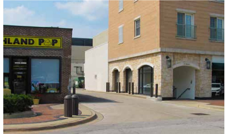
Service and Loading Access. Access to service and loading area off alley along Second Street
