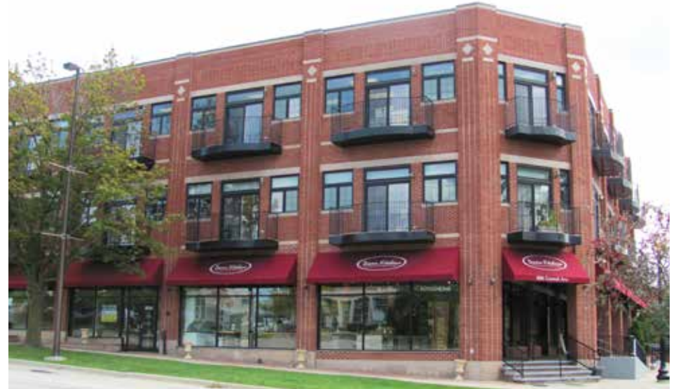
Building Material and Facade Example. Building along Central Avenue
