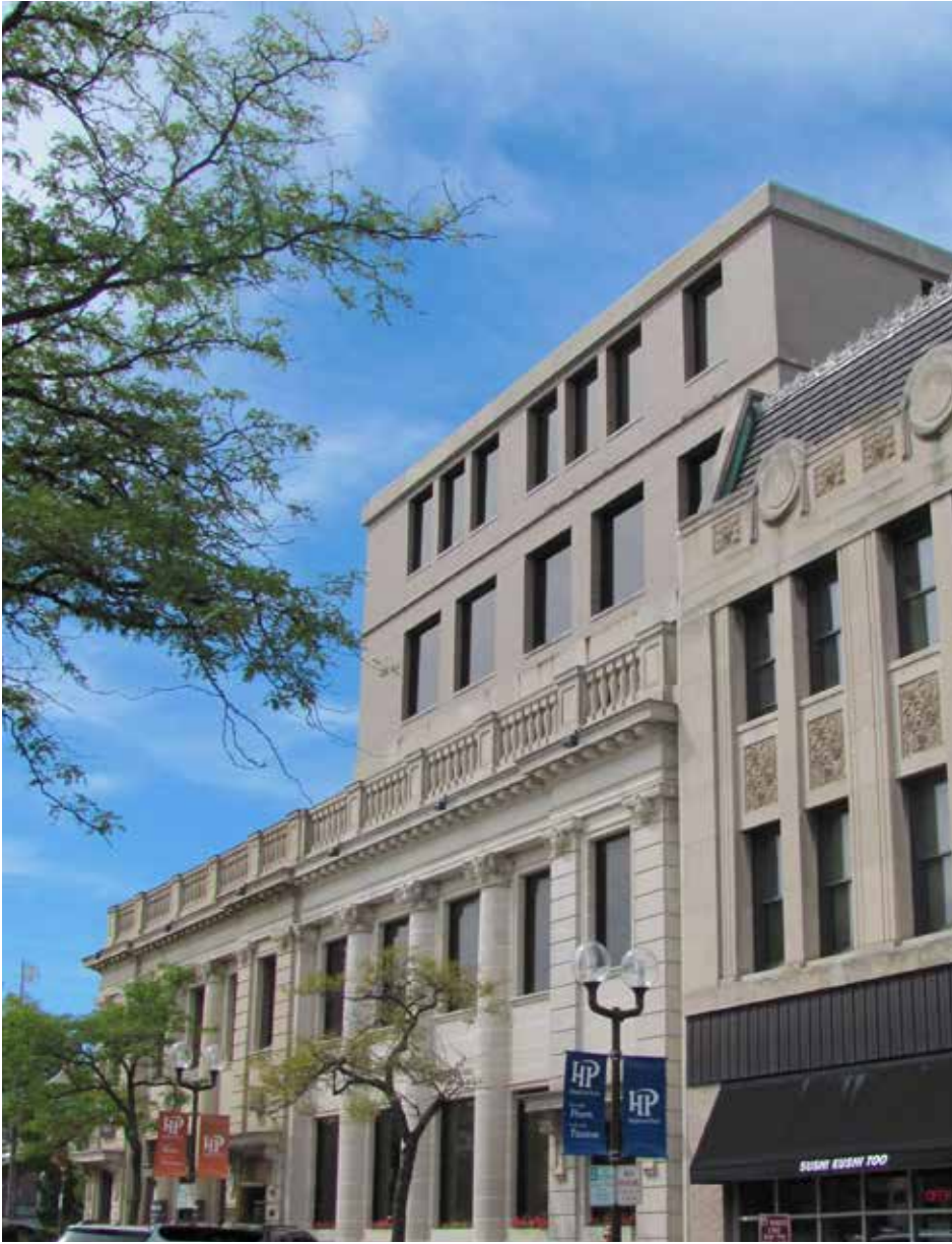
Height Step Back. Upper stories of building are stepped back away from the public right-of-way along Central Avenue
