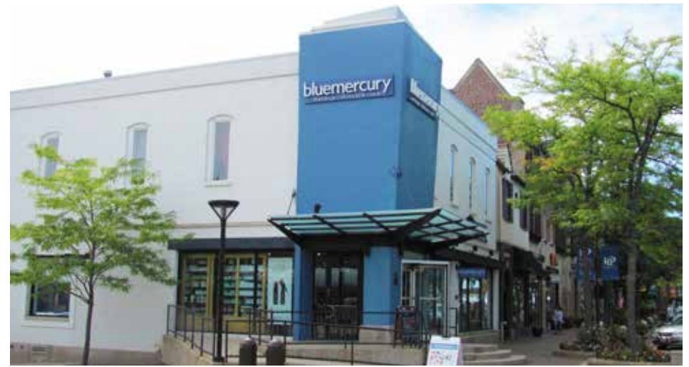
Corner Lot. Building design takes advantage lot at the corner of Central Avenue and Second Street with glass canopy and change in exterior building material color
