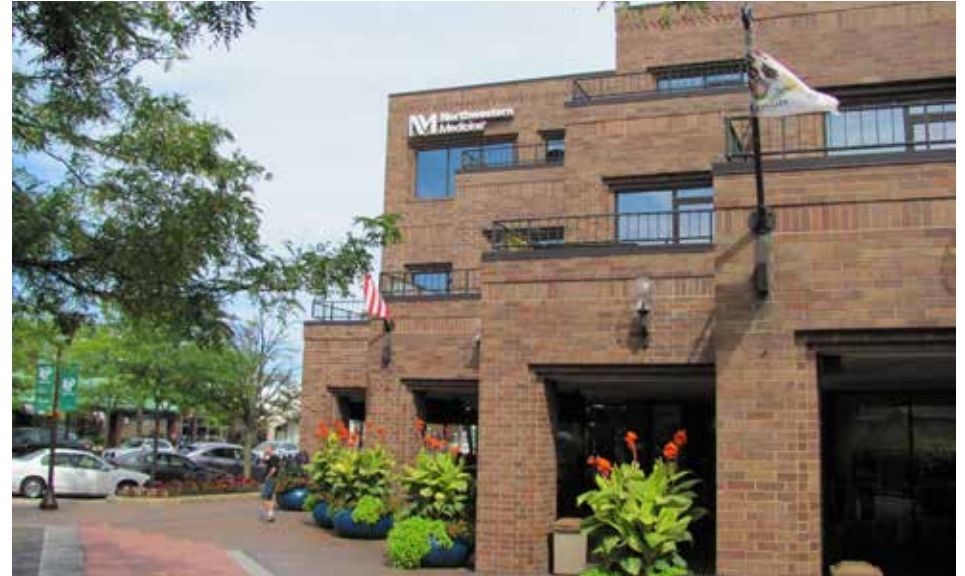
Height Step Back. Port Clinton building height step backs back from the pedestrian plaza and along Central Avenue
