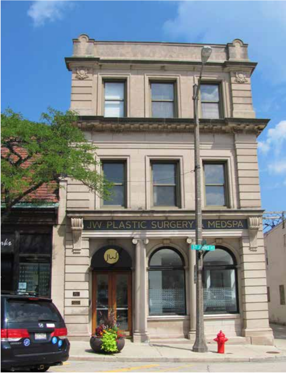
Building Material and Facade Example. Building along St. Johns Avenue
