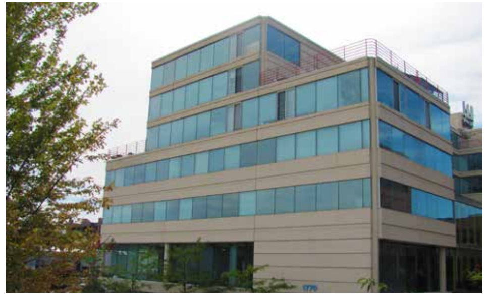
Height Step Back. Building height steps back from public right-of-way along Laurel Avenue
