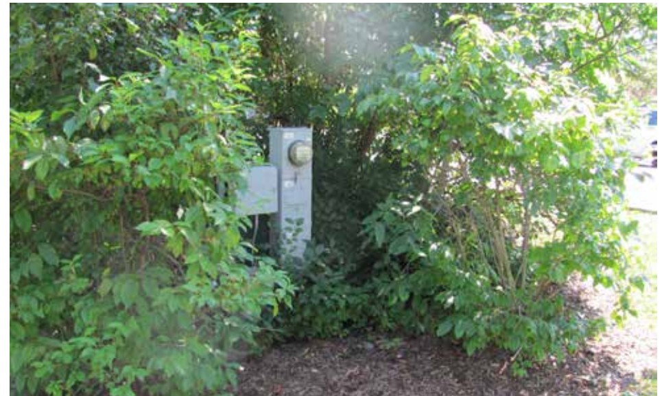
Mechanical Screening. Equipment is screened with landscaping along St. Johns Avenue in the Ravinia district
