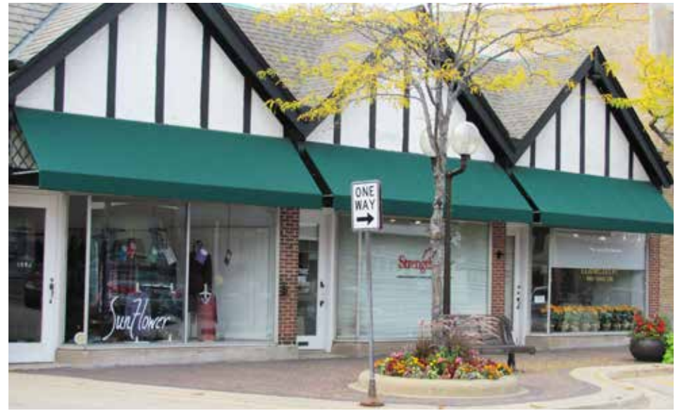
Awnings. Awnings on building along of Sheridan Road
