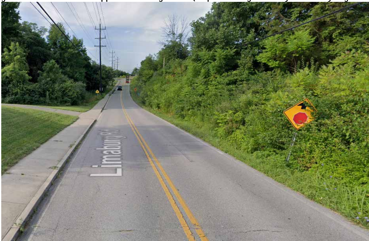
Figure A1-16: Southbound Approach to Cougar Path (Stop Ahead Sign Partially blocked by Vegetation)
