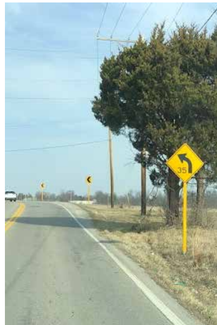
Figure 10: W1-1a Used as Advanced Warning Sign
