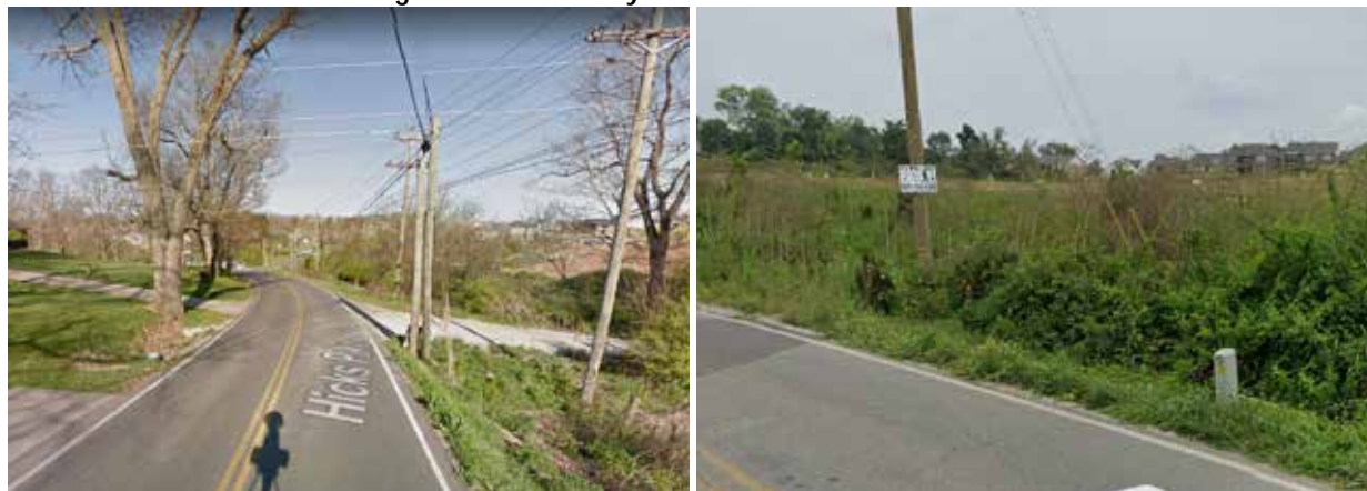
Figure A6-12: Utility Pole Locations on Hicks Pike
