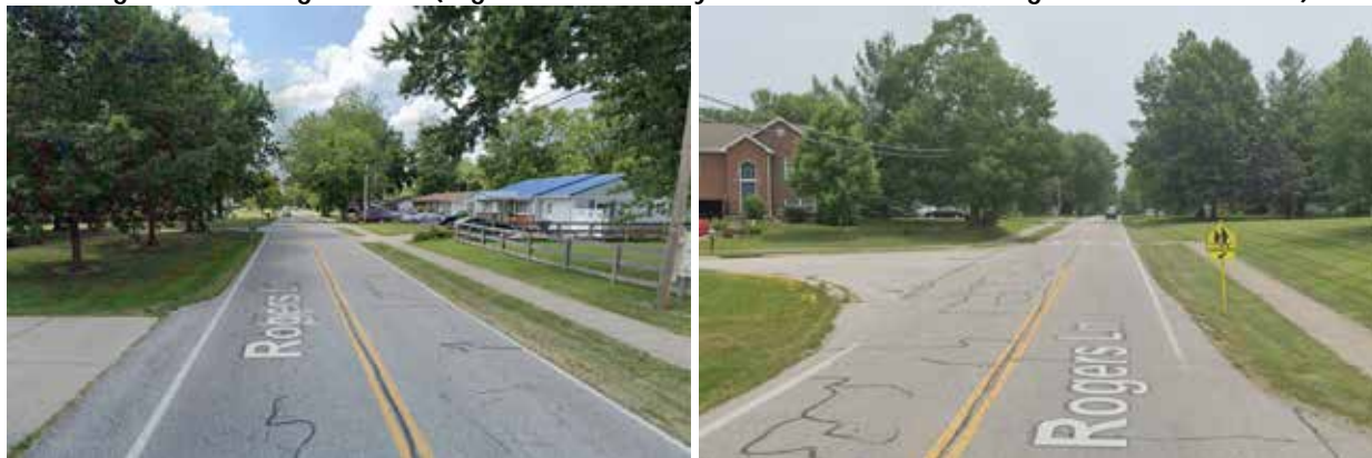
Figure A3-5: Rogers Lane (High Access Density and Pedestrian Crossings South of Utz Lane)
