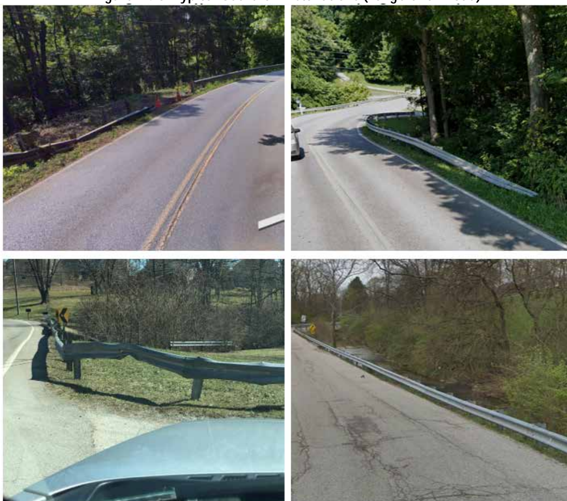
Figure A4-5: Typical Guardrail Installations (Longbranch Road)
