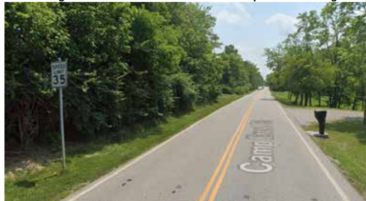
Figure A2-11: Left Side Mounted Speed Limit Sign
