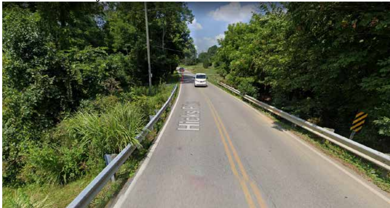
Figure A6-7: Culvert on Hicks Pike west of Harrison Road.
