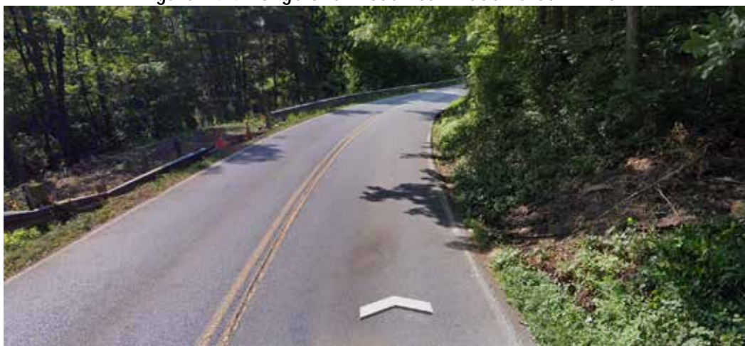
Figure A4-4: Longbranch Road near Hidden Creek Drive
