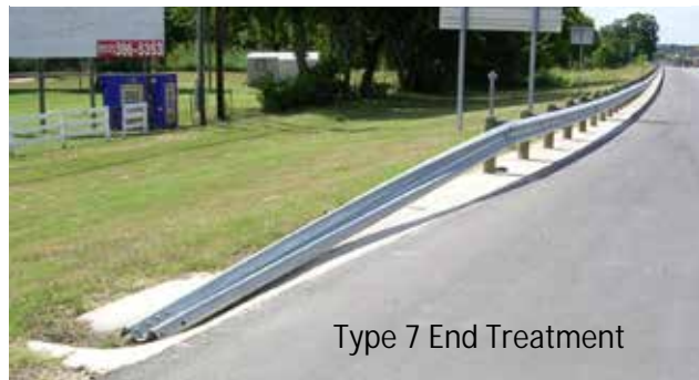
Figure 24: Type 7 End Treatments
