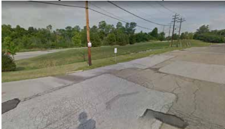
Figure A9-5: Drainage Ditch between Florence Square and Retail Access
