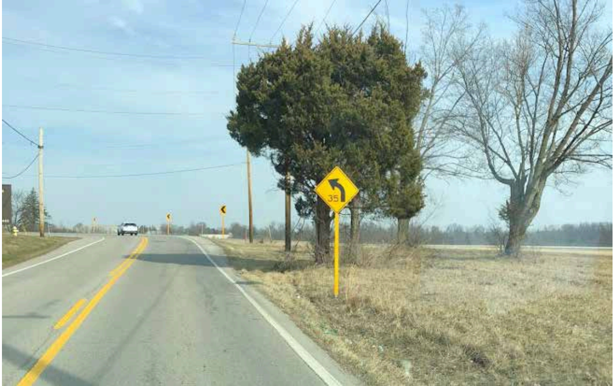
Figure A1-5: Horizontal Alignment Signing (Limaburg Road)
