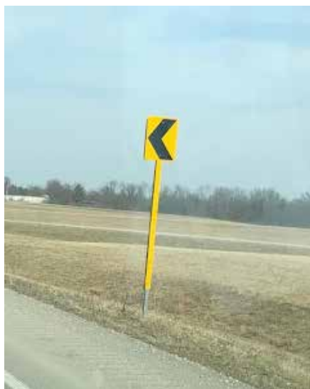
Figure A1-8: Horizontal Alignment Chevron
