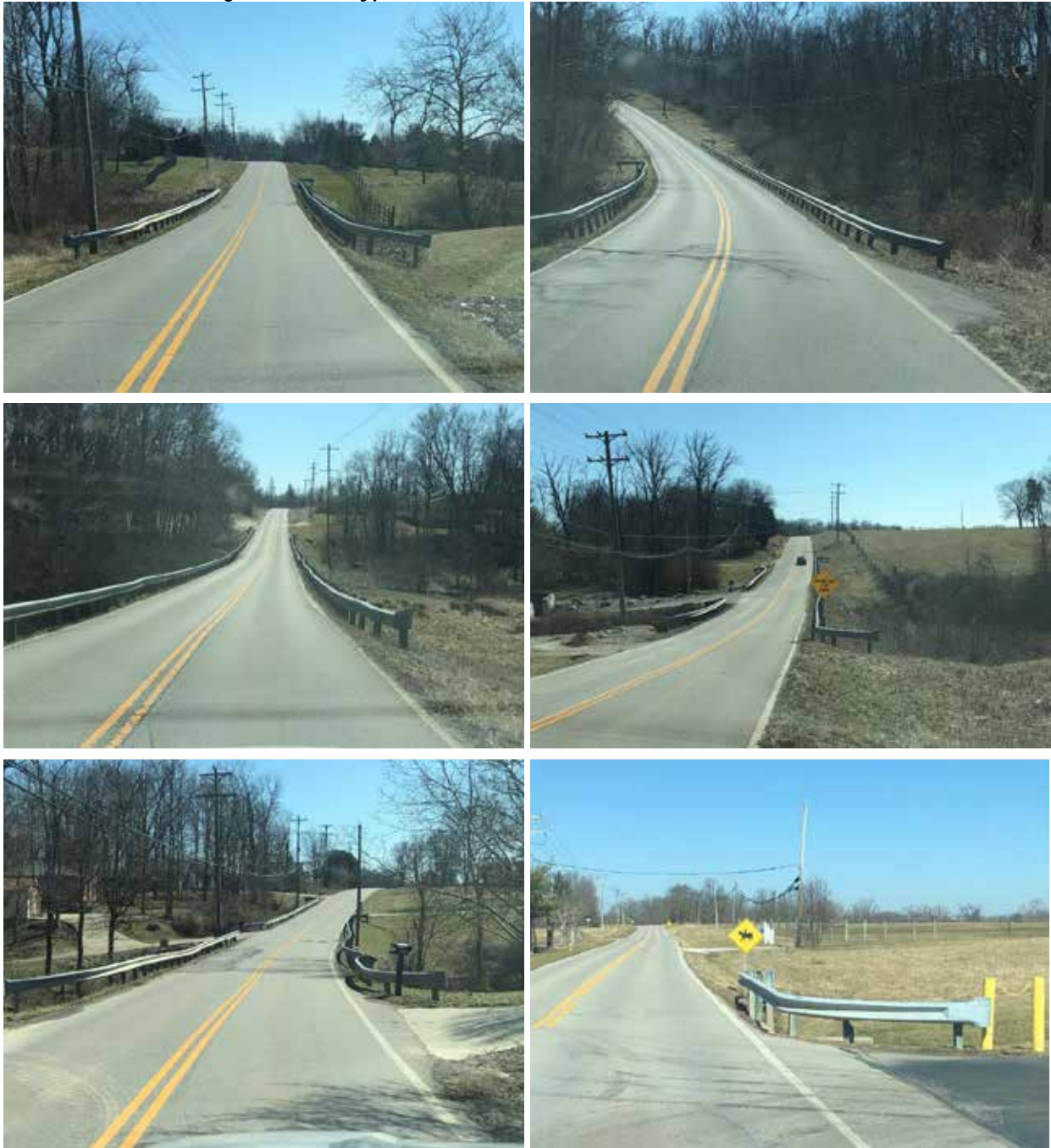
Figure A8-13: Typical Guardrail Installations on Bullitsville Road
