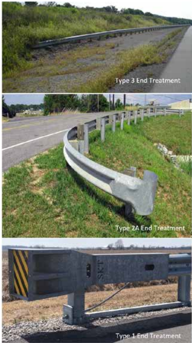
Figure 23: Preferred Guardrail End Treatments
