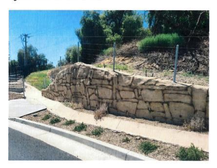
Figure 2. Boulder Face Soil Nail Wall
