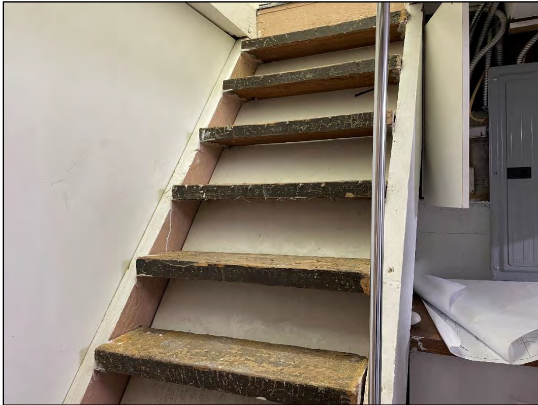
Figure 31. Detail view of the basement stairs.
