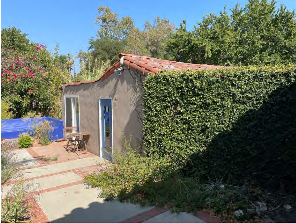
Photo 7. Northwest façade of the garage, view to the east.
