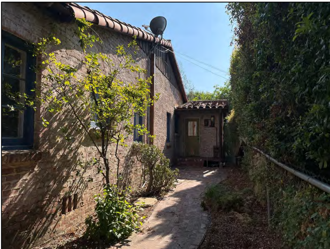
Figure 20. View of the porch and exit on the northeast façade of the maid's quarters.
