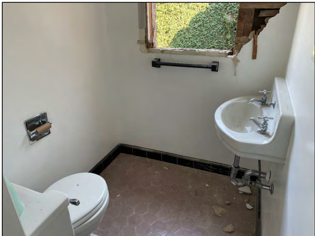
Figure 32. Interior overview of the half-bath.
