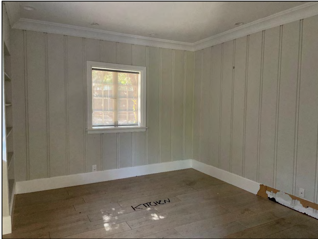
Figure 23. Interior view of the library, looking west.
