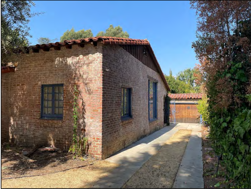
Figure 13. View of the southeast façade of the main wing, looking north.
