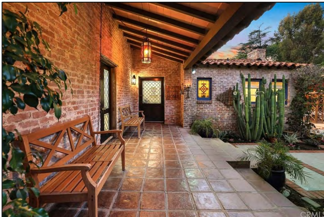
Figure 16. Overview of the concrete porch and southeast façade of the secondary wing prior to removal of doors, windows, and tiles (Redfin 2020).
