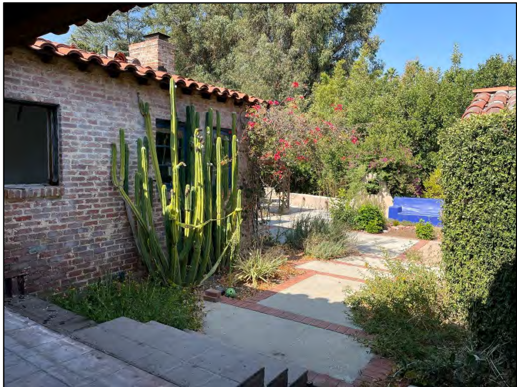
Figure 14. Partial view of the southeast façade of the secondary wing and rear yard, looking northwest.
