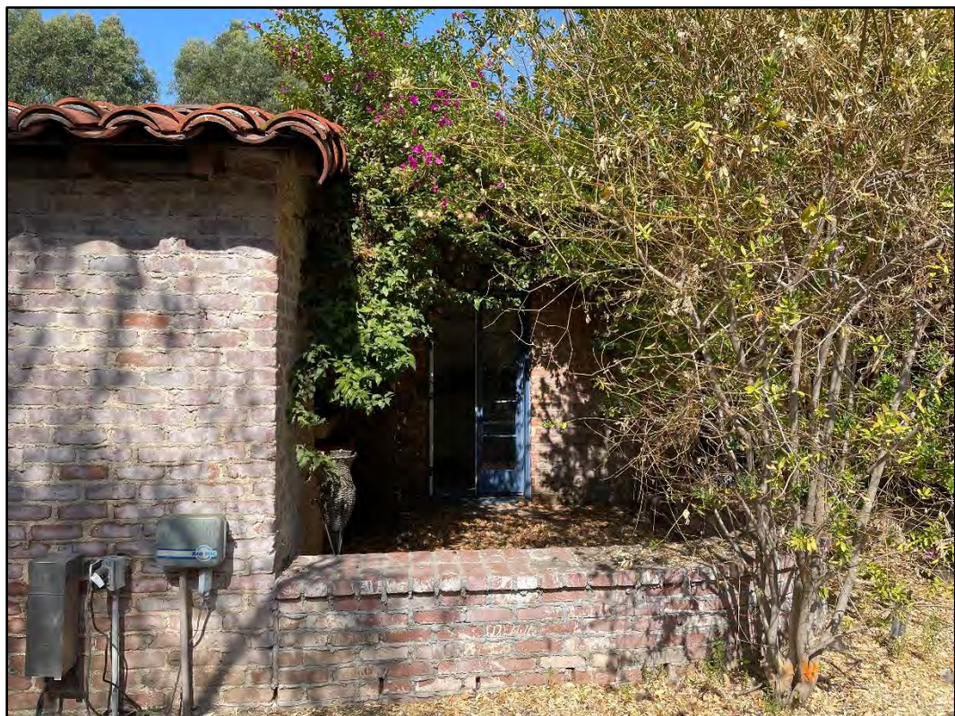
Figure 12. Overview of southwest patio and French door entrance, looking northeast.
