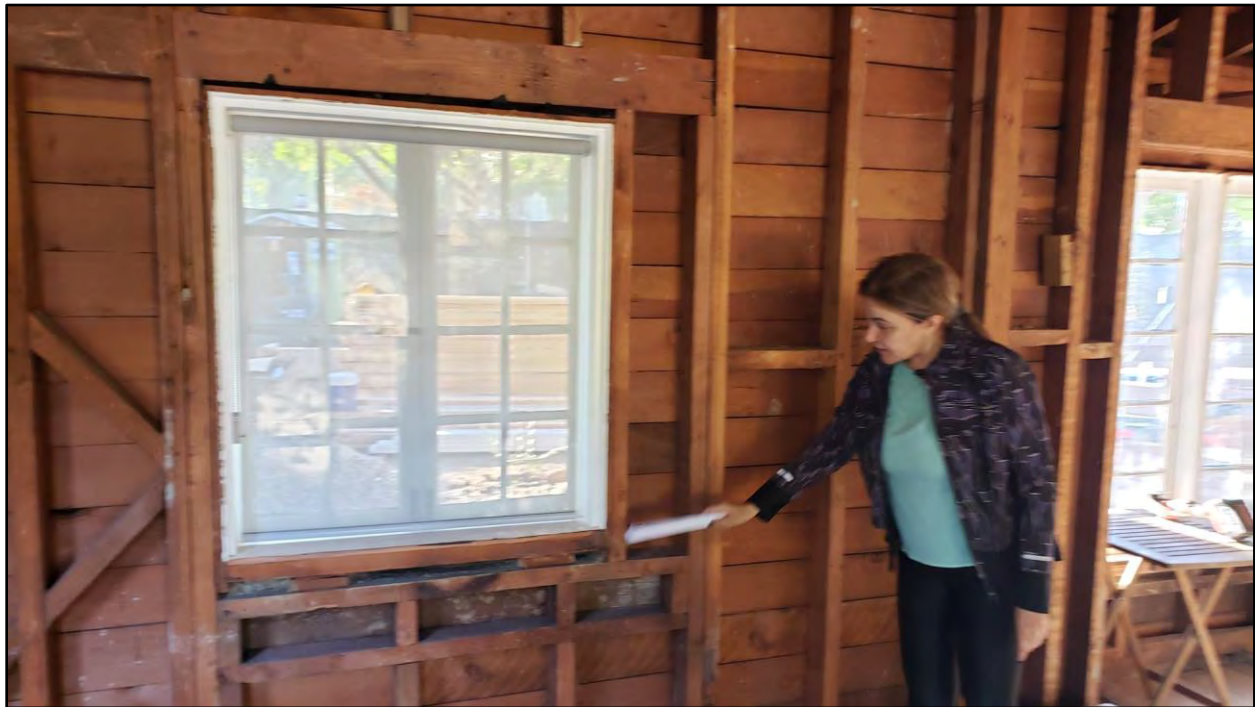
Figure 38. Interior wall construction of W01 showing original, larger size.
