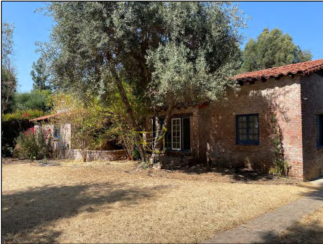
Figure 11. Overview of the west façade, looking north.
