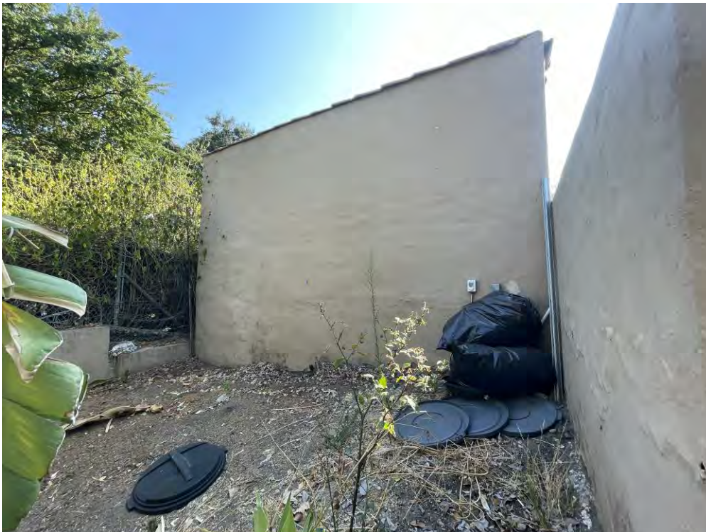
Photo 8. Northeast façade of the garage, view to the south.
