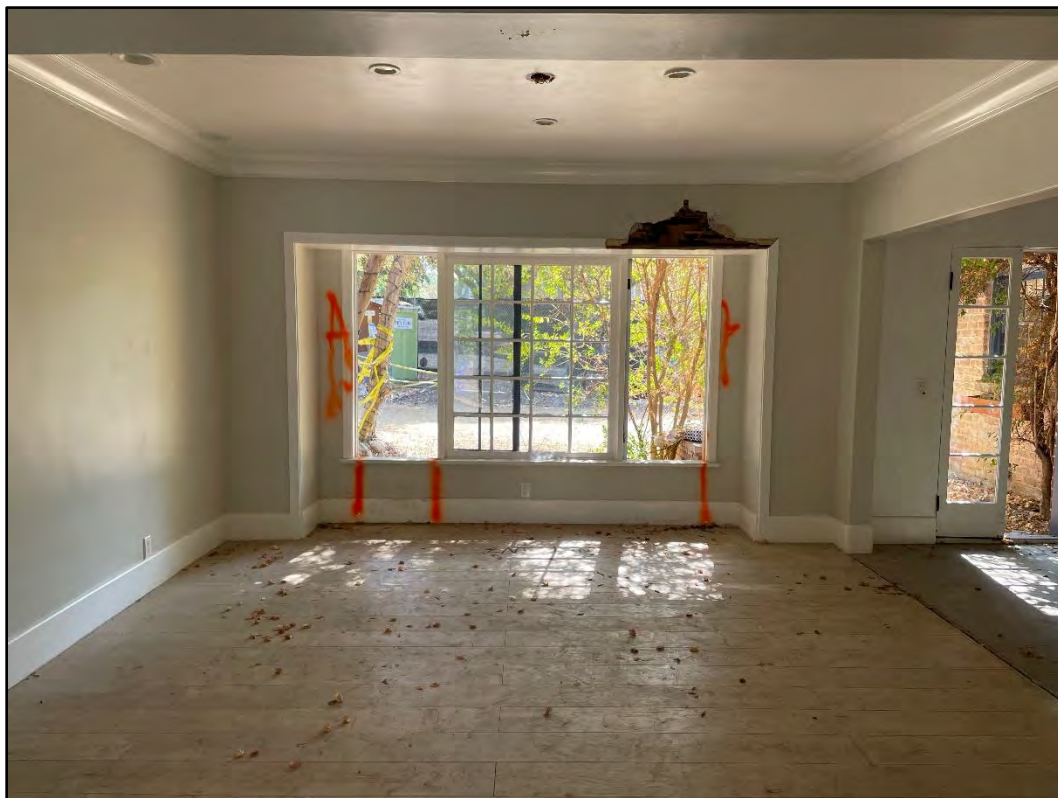
Figure 22. Interior overview of the dining room looking west.
