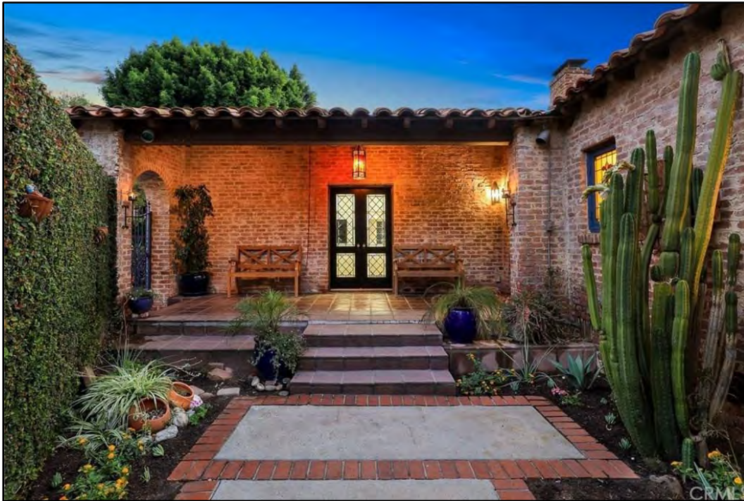
Figure 17. Overview of the concrete porch and northeast façade of the main wing prior to removal of doors, windows, and tiles (Redfin 2020).
