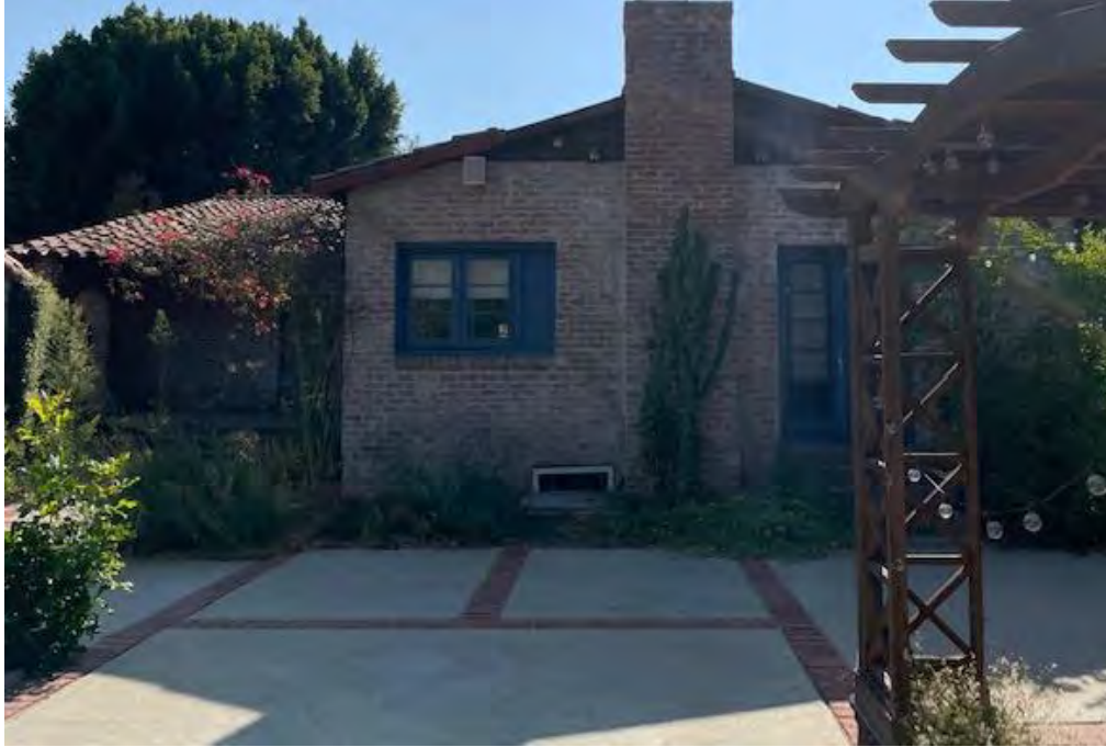
Photo 5. East façade of the residence, view to the northeast from the upper rear yard.
