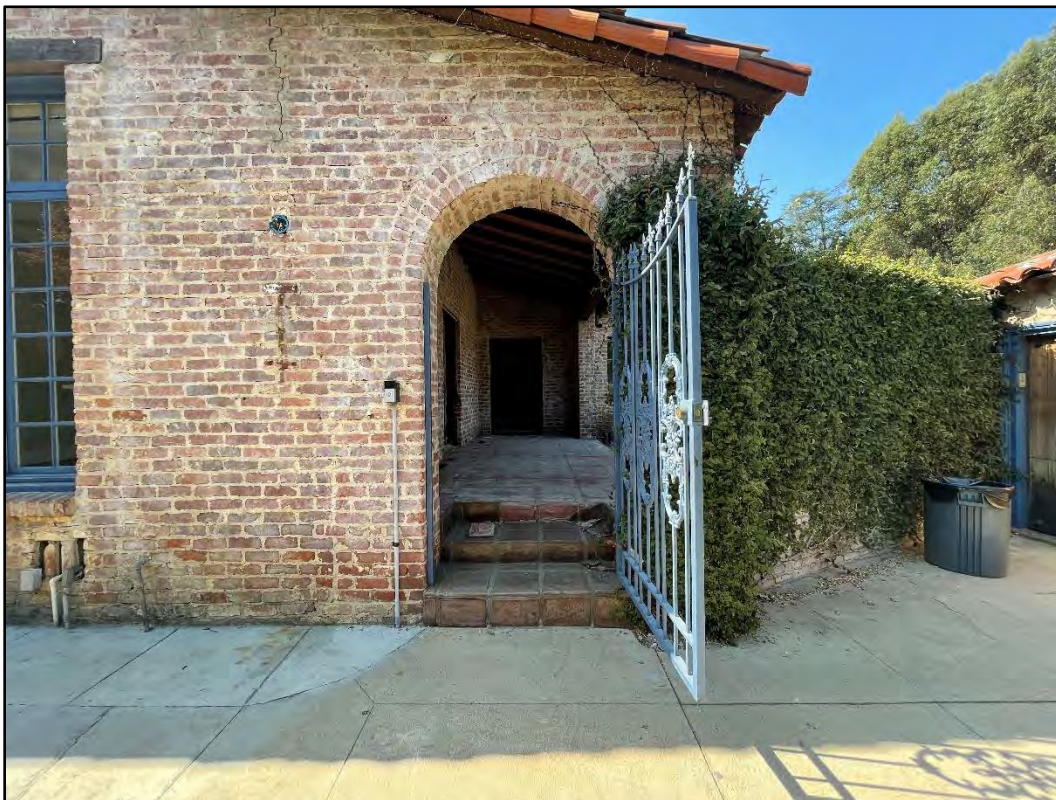
Figure 10. View of southeast porch entrance, looking northwest.
