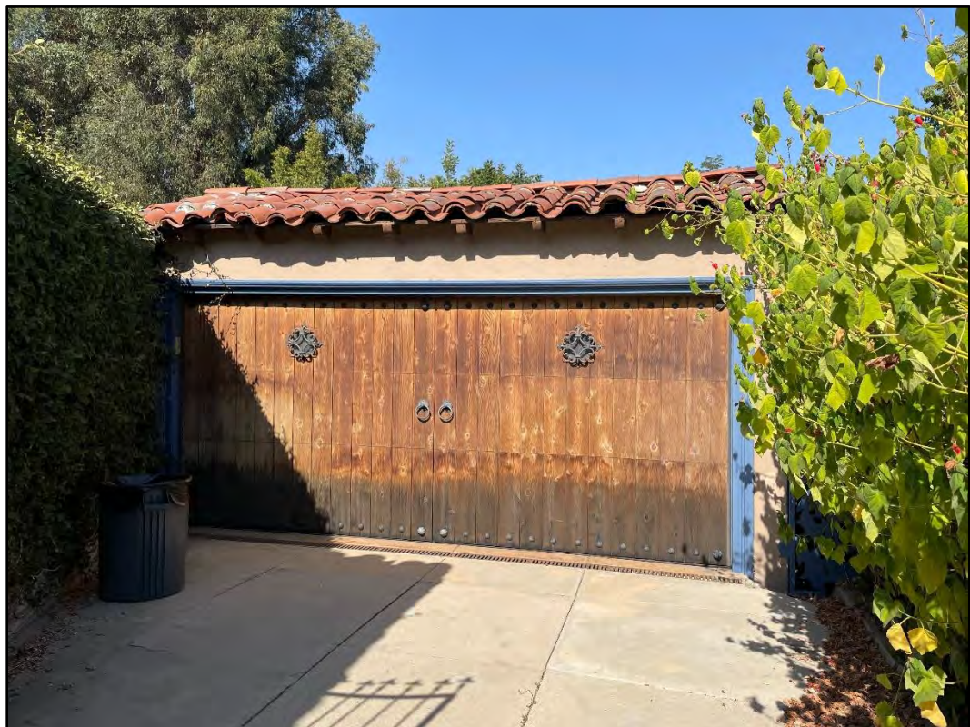
Figure 8. Overview of the garage, facing northeast.
