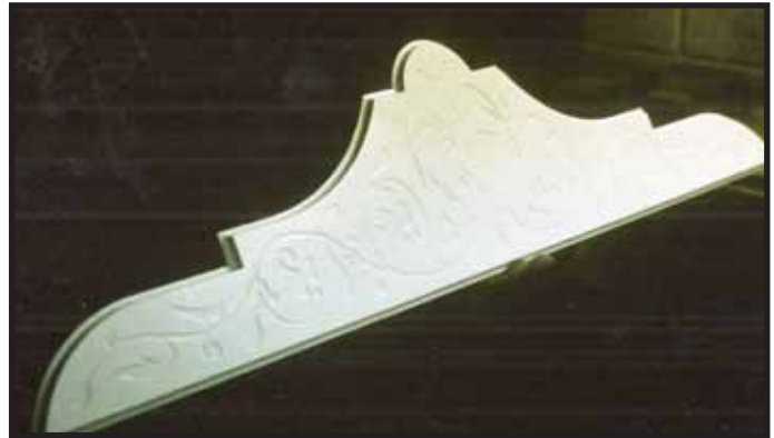
Figure 37. Assembled with added scroll design, the new crown is primed and ready for finish painting.
