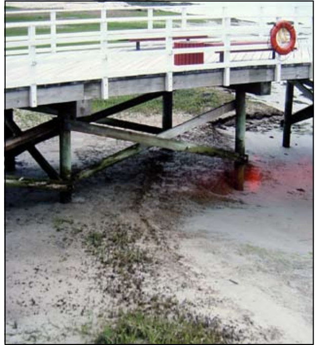
If docks are not designed to minimize shading, they will lead to marsh loss much greater in area than their actual footprint. Photo Michele Dionne.
