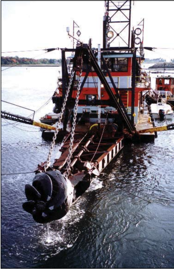
Dredge equipment in the Webhannet Harbor, year 2000. Photo Susan Bickford.
