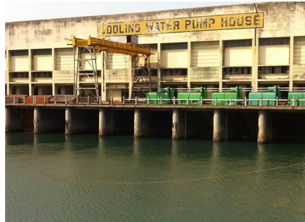
Station 3 (1 st Stage Intake)
