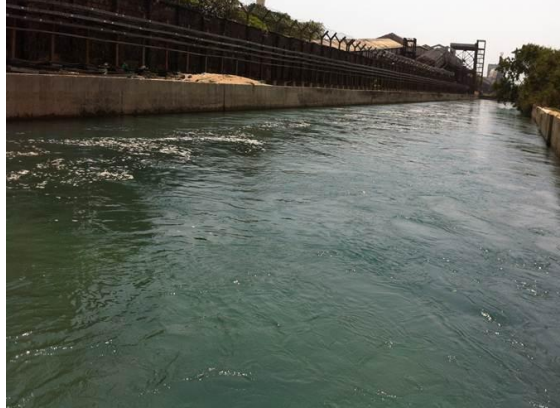
Station 7 (II nd Stage outlet located on inlet channel)
