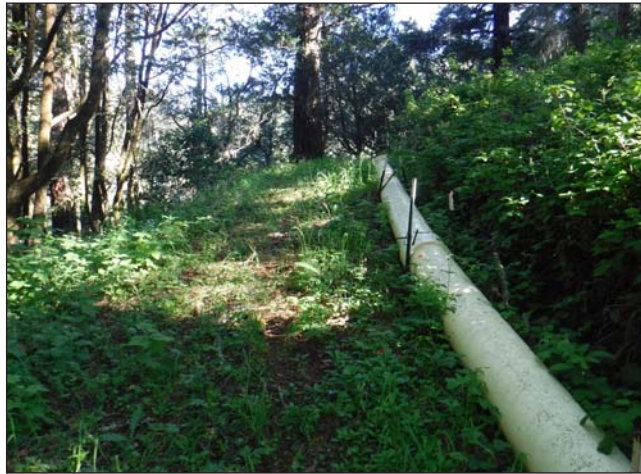
PHOTO 1: Representative pipeline corridor in southern part of study area.
