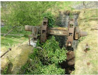
Slide 85 28 foot wheelpit, with axle in situ, this is the wheel that wound No 3 Shaft.
