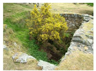
Slide 68 One of the two semi-circular ore bins, before clearance
