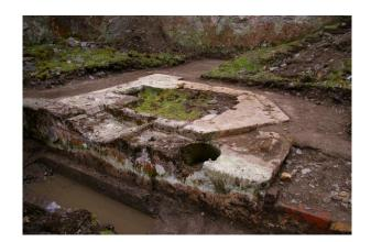
Slide 32 Base of Pelton Wheel with water drain on the right
