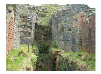
The wheelpit contained a 40 foot iron waterwheel as opposed to the normal wooden variety. This wheel was purchased from the Oola Mine, in Co Limerick, Ireland.
