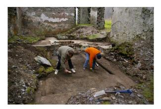
Slide 34 Base of Steam Engine and Alternator are uncovered
