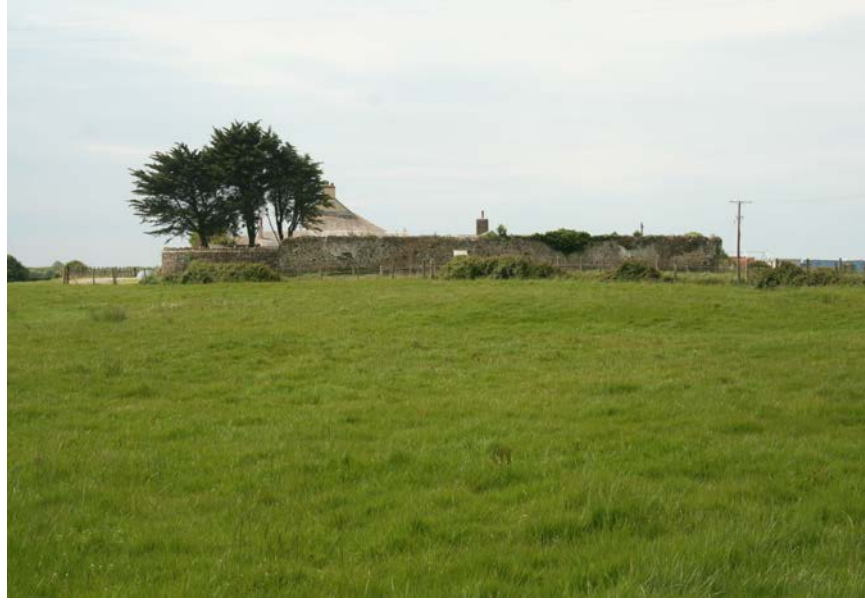
A2: Northern end of Hurst House boundary wall in north-western end of Area A (looking south)
