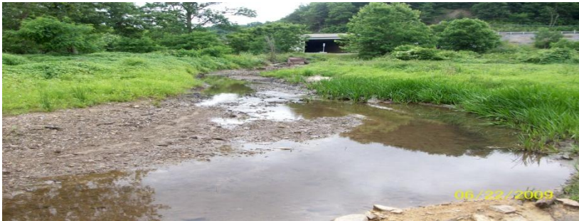
Site #7 – This is feeder stream that has broken through the dam and is carrying the legacy sediment around the dam and into the stream below.
