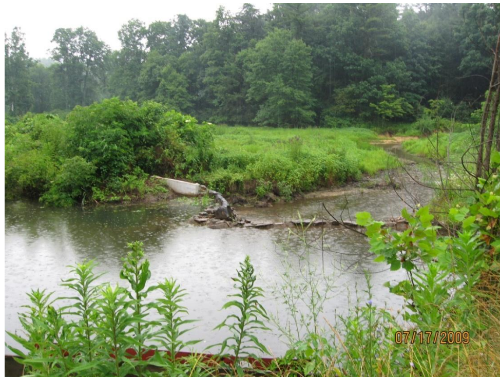
Photo 12. Looking at the current impoundment above the Burnt Cabins Grist Mill, with some flow running parallel to the impoundment and flowing over the spillway. The small dam in the foreground is a makeshift structure to facilitate the needed height for water to enter the gate valve at the top of the mill race (on which the photographer is standing)
