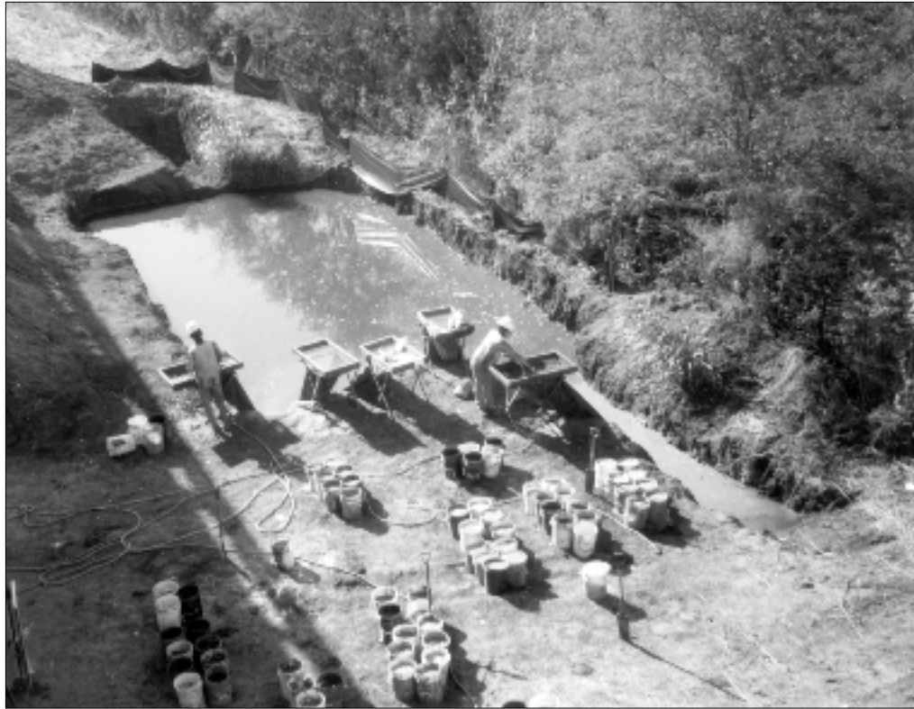
Figure 5-2. Water screening stations and settling pond.
