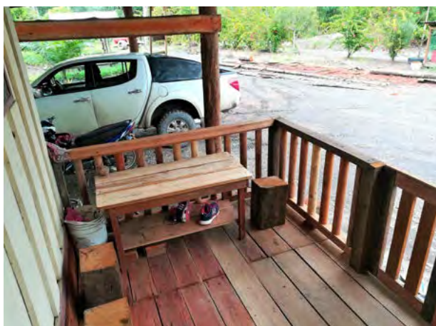
Deck and railing constructed using E. pellita timber; Sarawak, Malaysia (Photo: R. Arnold)
