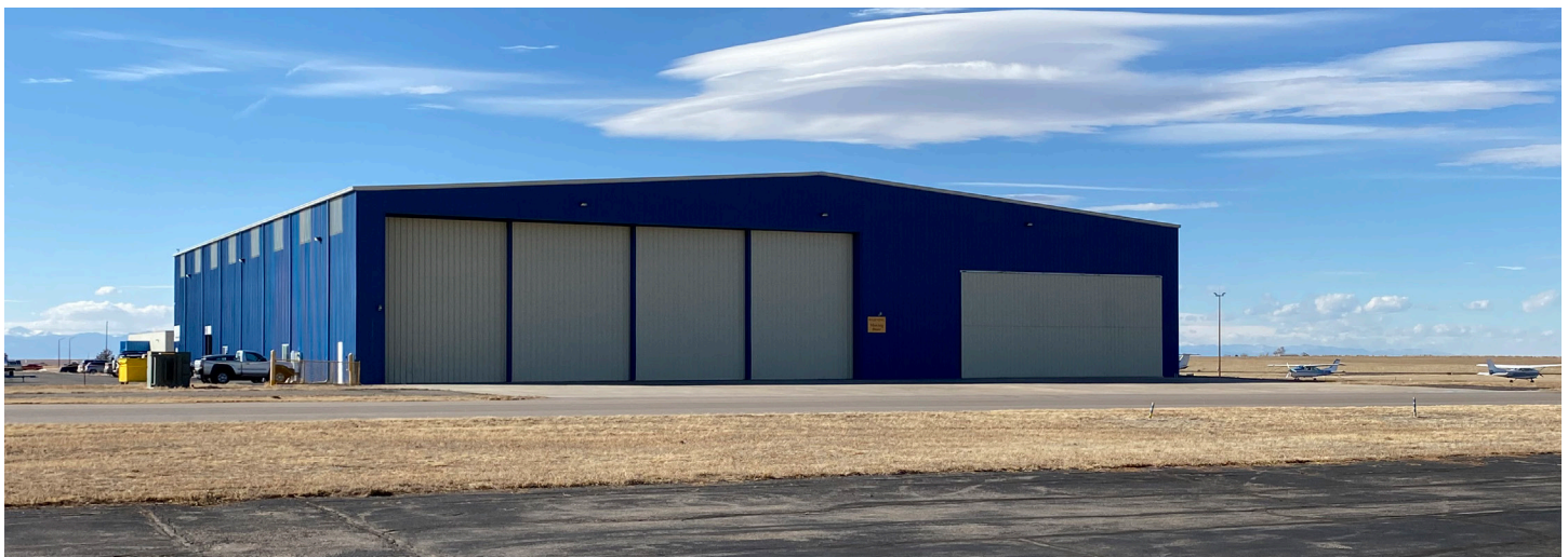
Figure 4-7. Private Hangar at Colorado Air and Space Port
