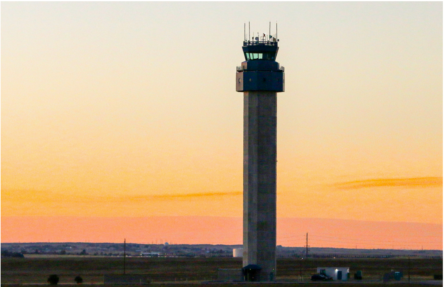
Figure 4-8. CASP Air Traffic Control Tower
