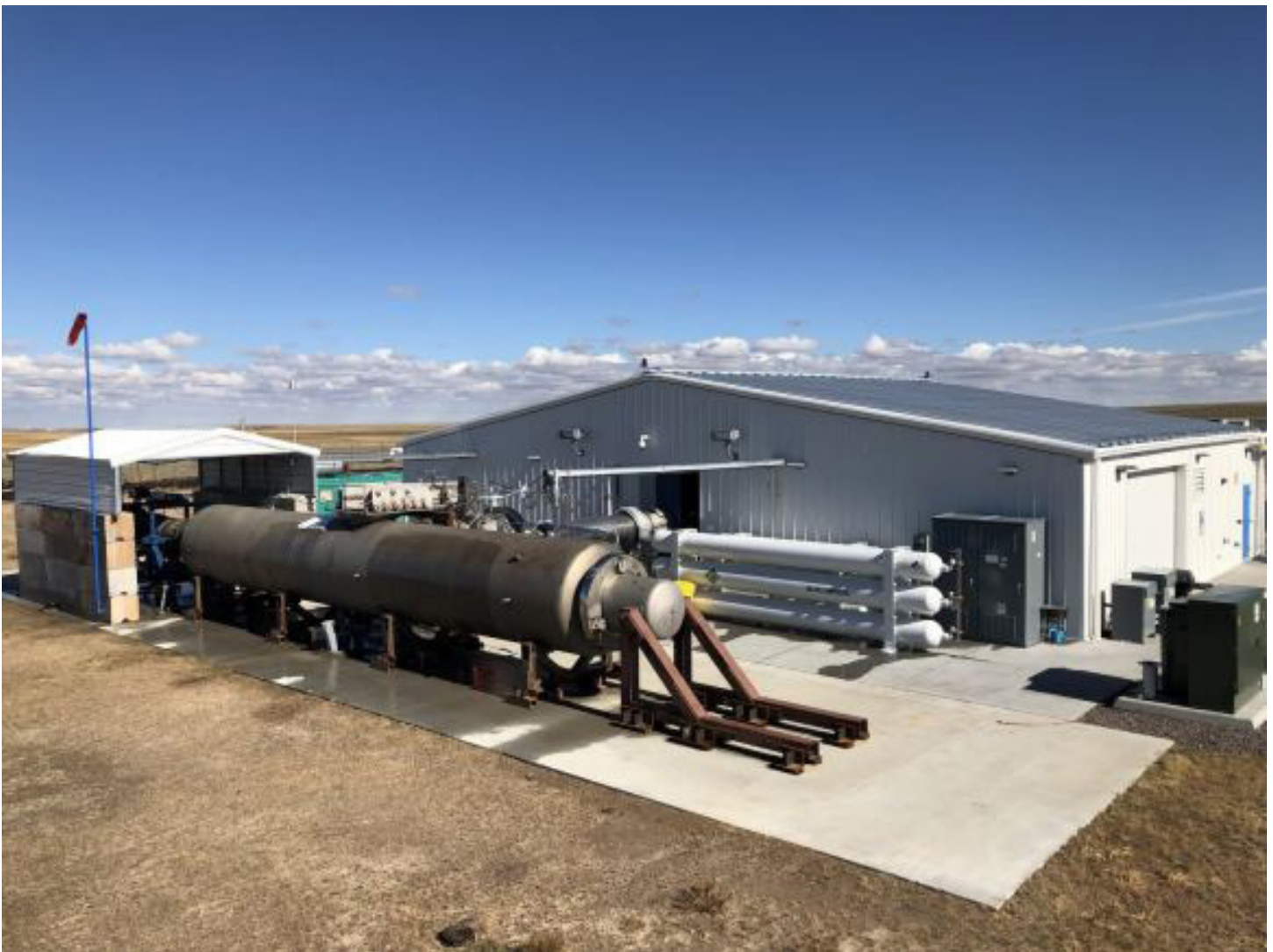
Figure 2-5. Reaction Engines Test Facility 2
