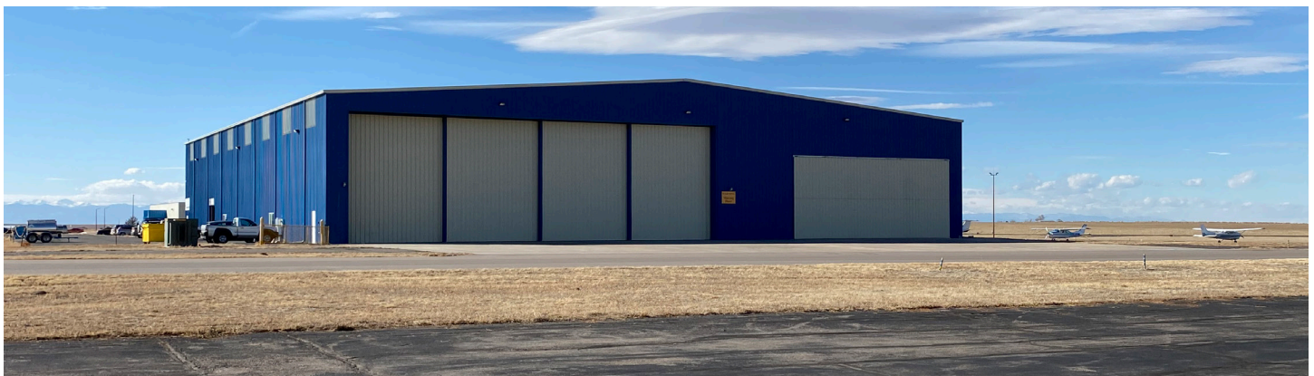
Figure 5-8. Existing Hangers at CASP
