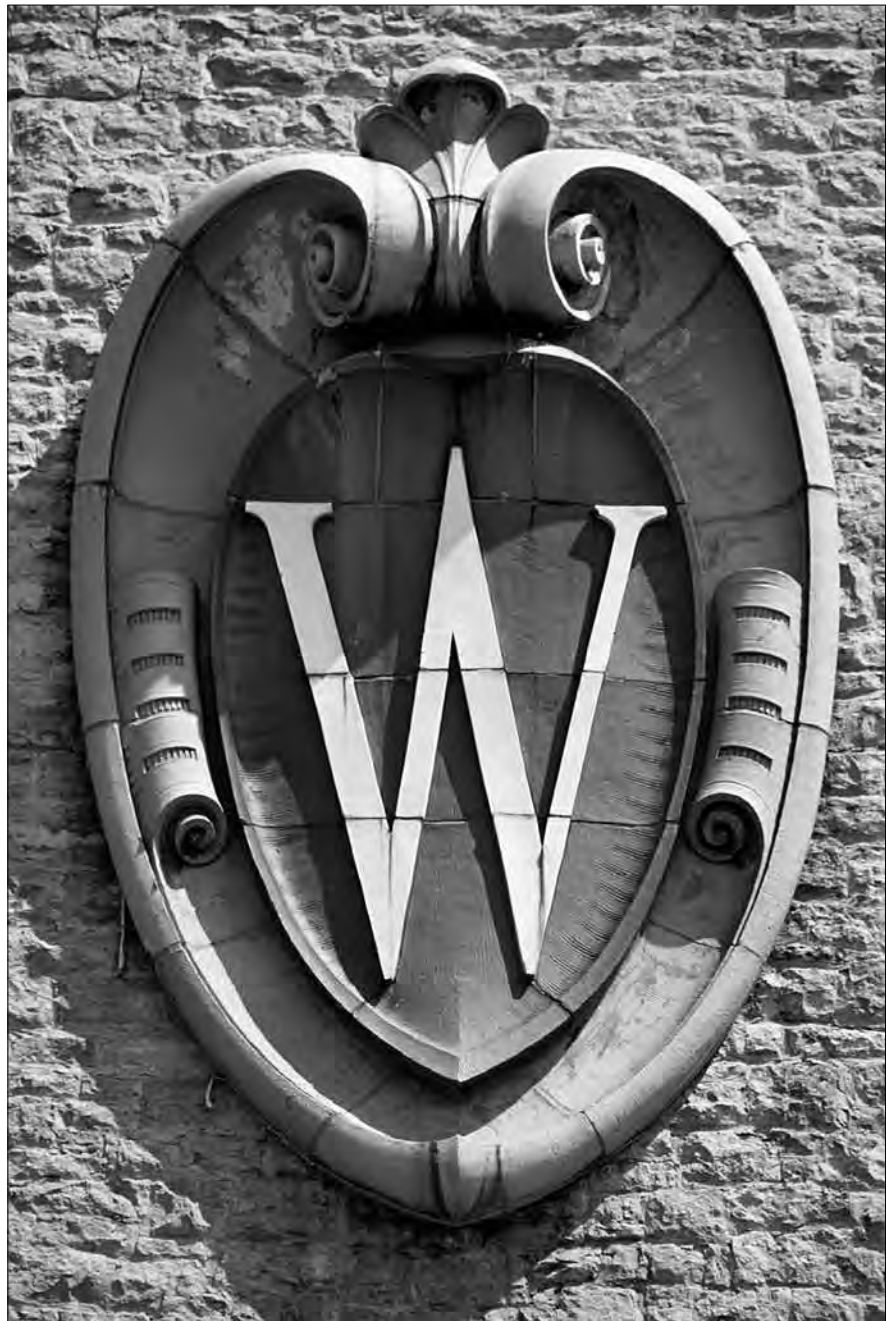
Architectural detail, UW Field House
