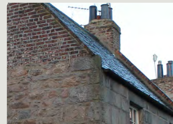
Figure 5.58: Reclaimed granite and brick gable
