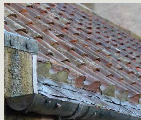
Figure 5.57: Traditional eave detail
