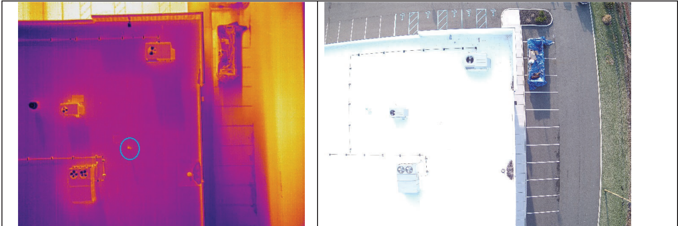
Area 1 – Exhaust pipe – No Concerns
