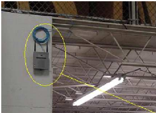
Figure D-3 AP and Antennas Mounted on a Wall, Away from I-Beams
