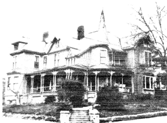
The "Governor's Mansion," which stood at the corner of Fourth Ave. and Gill St., was built for former Tennessee governor and senator Robert L. Taylor in the late 1800's. The house was in decline for decades, and was not able to be saved before it burned down in the 1980's.
