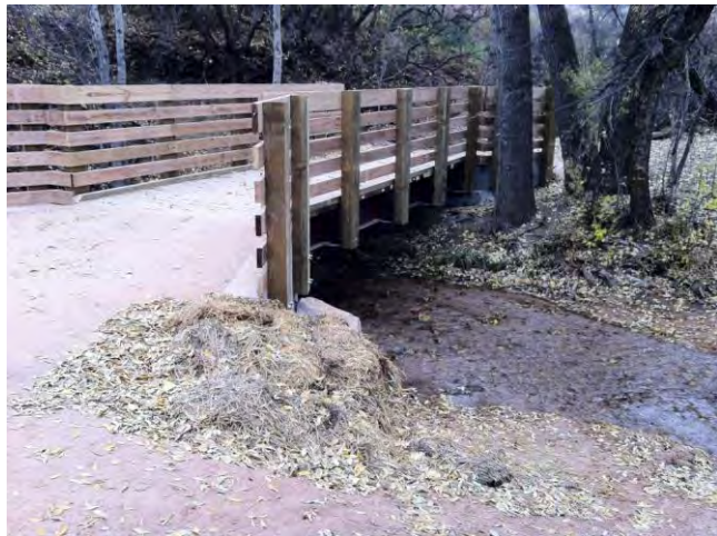
Pedestrian bridge across creek protects aquatic habitat
