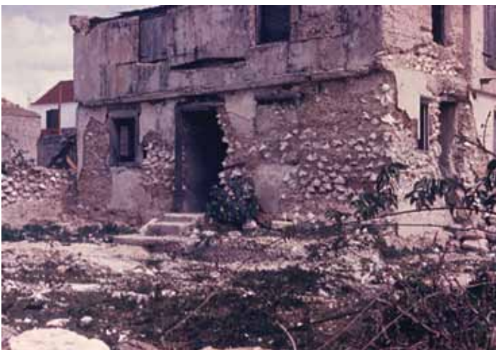
House incorporating Strombus gigas shells, Cockburn Harbor, South Caicos, Turks and Caicos Islands, January 1968. Photo by G.F. Quinby.
