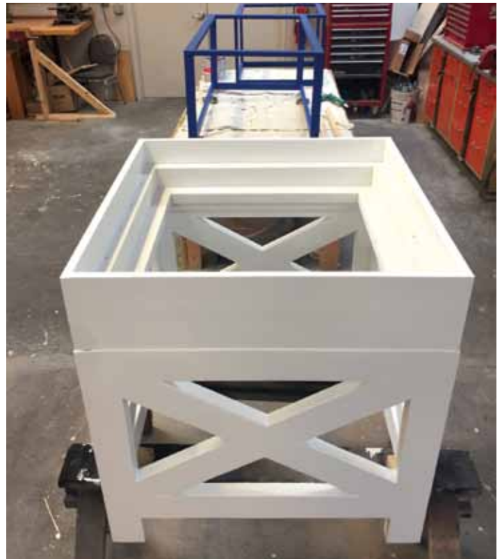
(Above): Stands and metal frames under construction.
