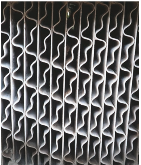
Preheater Basket After Cleaning with NitroLance
