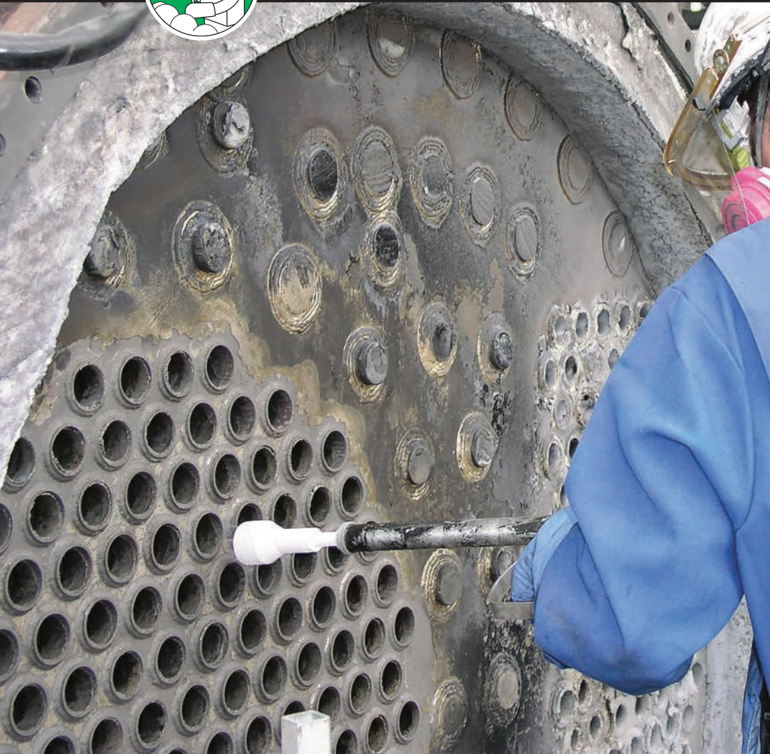
0.320" Thick Hardened Carbon Based Deposit
