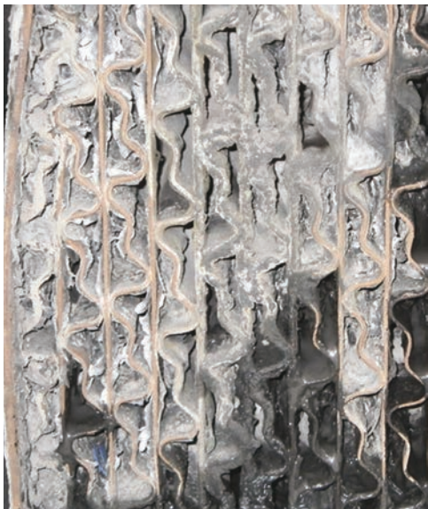
Preheater Basket Before Cleaning with NitroLance
