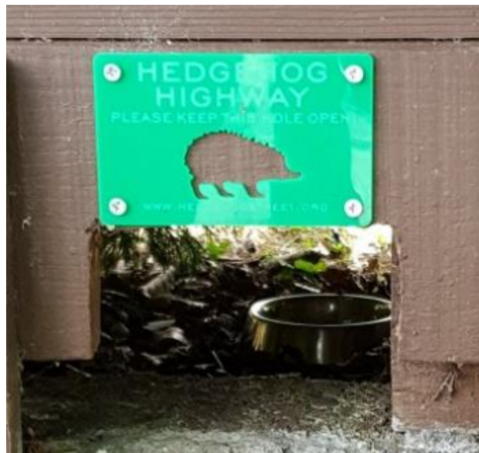
A sign explains the wall gaps
