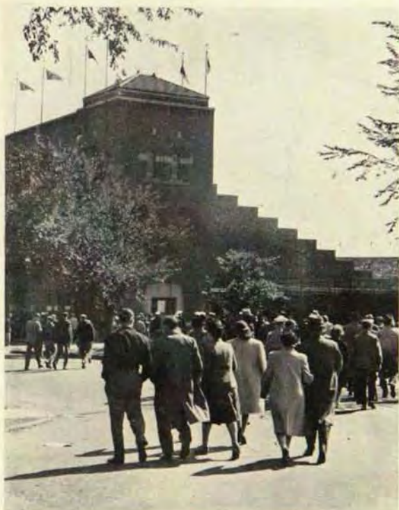
North Tower, Memorial Stadium
