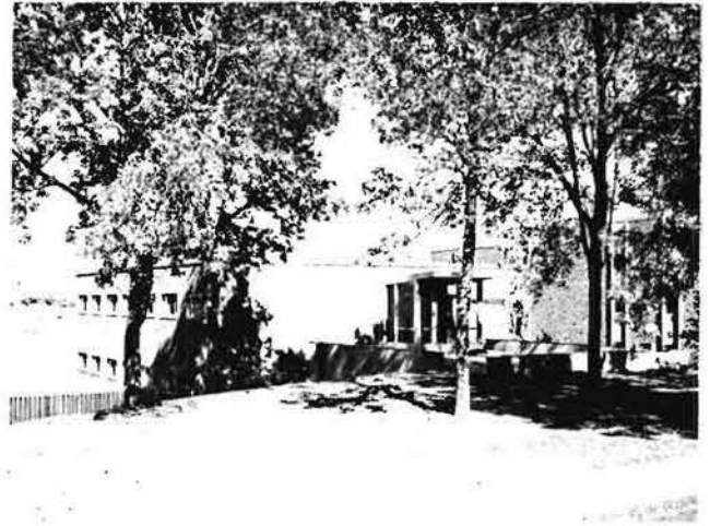
Forest Products Bldg
