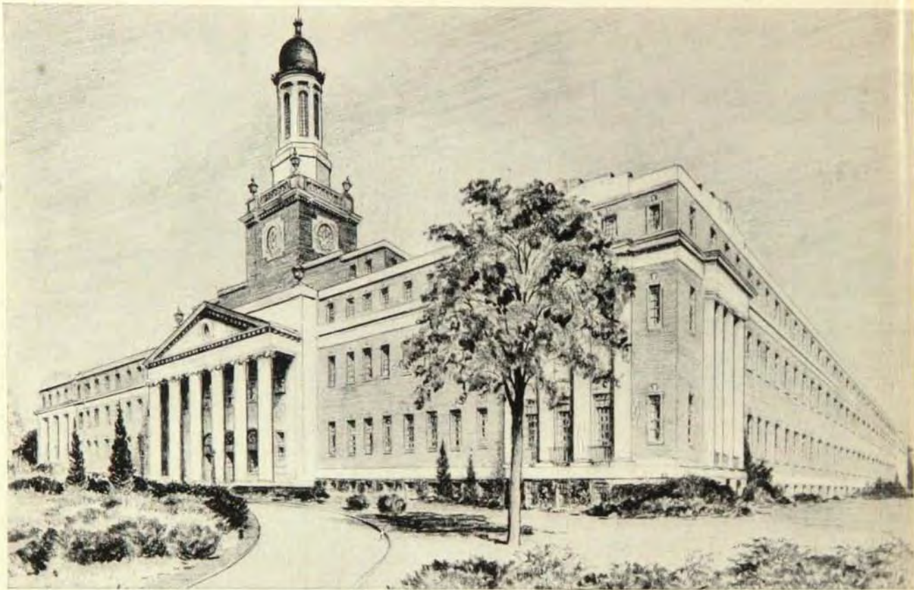
Massachusetts Mutual Home Office
