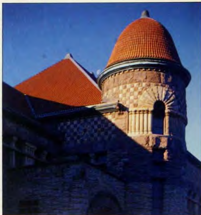
Pillsbury Hall's fanciful carving, varicolored stonework, and circular tower all play on Romanesque themes developed by architect Richardson.
