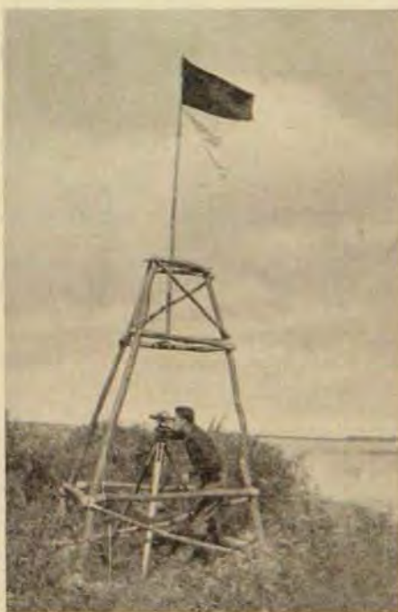
STRAWBERRY POINT SIGNAL TOWER One of the towers erected at the Engineers Surveying camp near Cass Lake to allow one party to read from station without interfering with others sighting this point.
