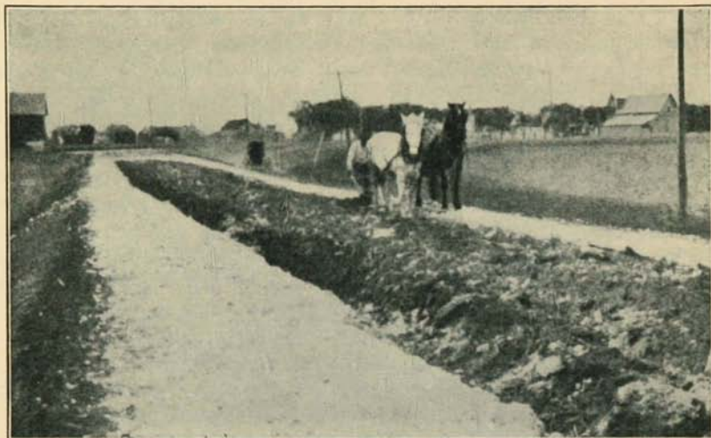
FIG. 1.—Marl being plowed into a sandy road bed, near Rice. (After Dow.)
