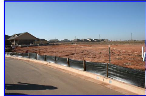
Figure 18. Silt fencing at construction site.
