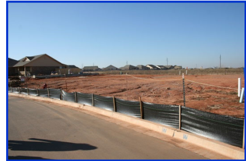
Figure 18. Silt fencing at construction site.
