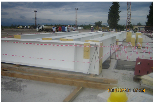
Fig. 4. The first assemblies arrive to building site on 01.07.2012
