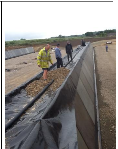
Laying impermeable membrane
