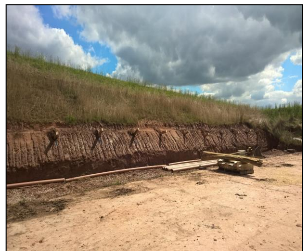
Earth banks being built up or 'dug in' prior to panel installation
