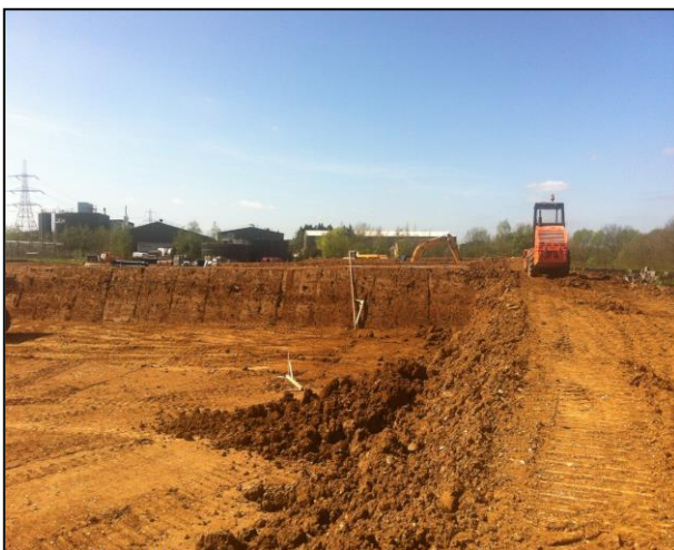
Earth banks being built up or 'dug in' prior to panel installation
